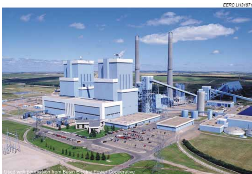
Figure 1 – Antelope Valley Station, near Beulah, North Dakota.
