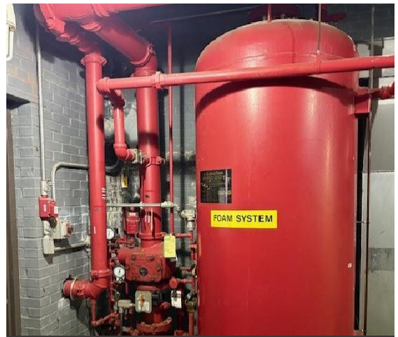
Photo 3.2.2.12: B-64 & B-92 Aqueous Film Forming Foam (AFFF) Fire Suppression System Replacement.
