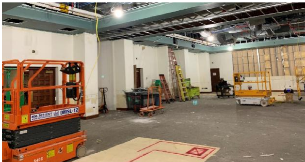
Photo 3.2.2.2a: B-922 conference center — room 106 before renovation.
