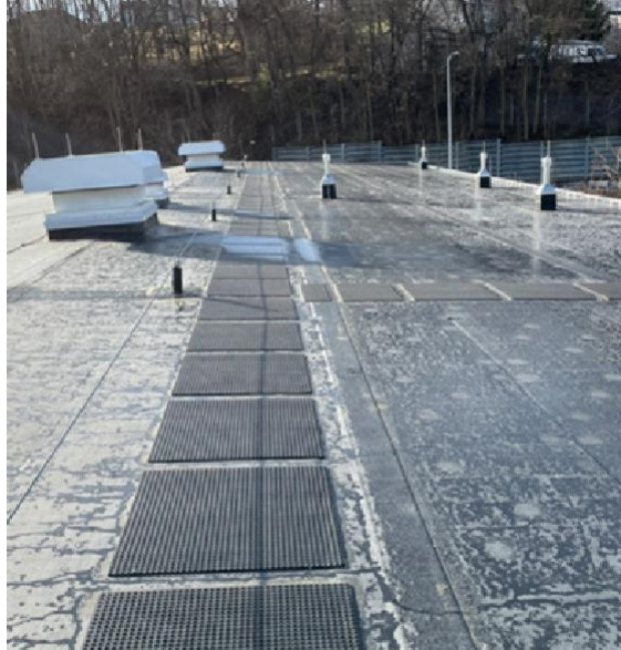
Photo 3.2.2.6b: B-901 — new roof with fall protection and lighting protection system.
