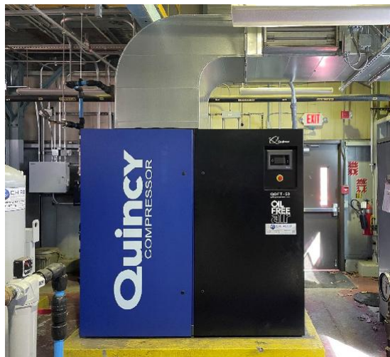
Photo 3.2.2.9a: Newly installed Quincy air compressor.
