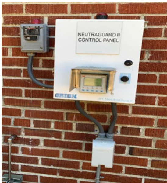
3.1.5.1.1a: Elementary neutralization system.
