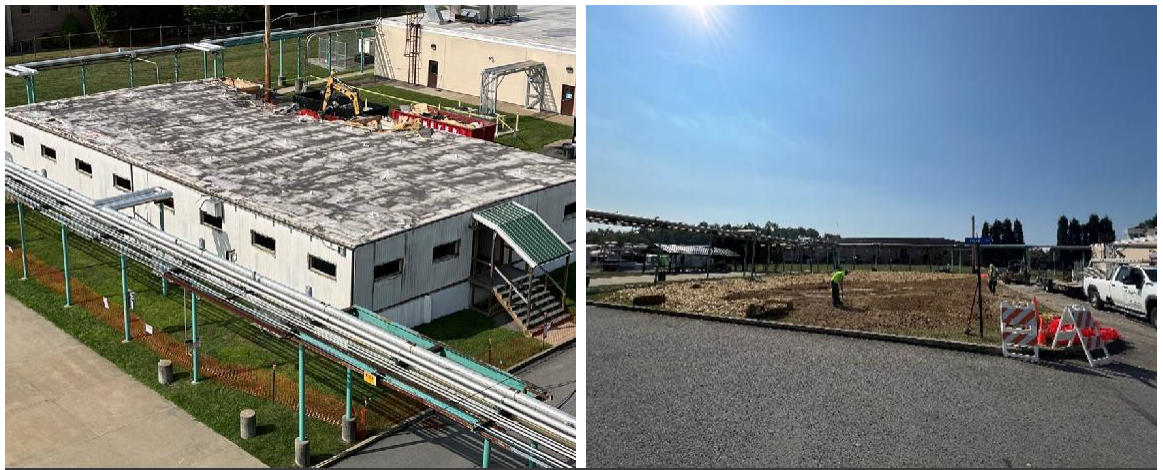
Photo 3.3.2.1: Trailer 40 before (left) and after demolition (right).
