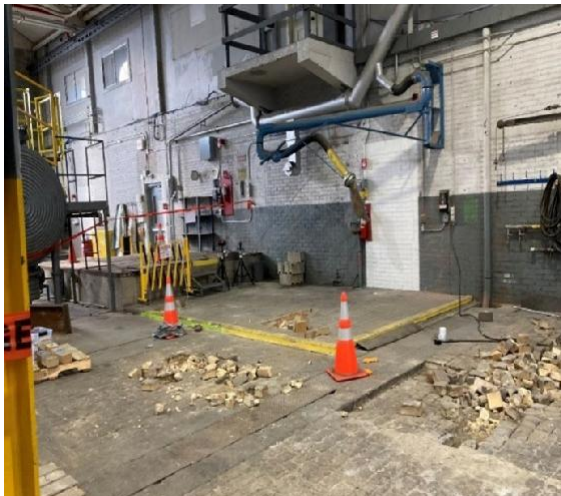
Photo 5.3.1a: Contaminated brick and sand.
