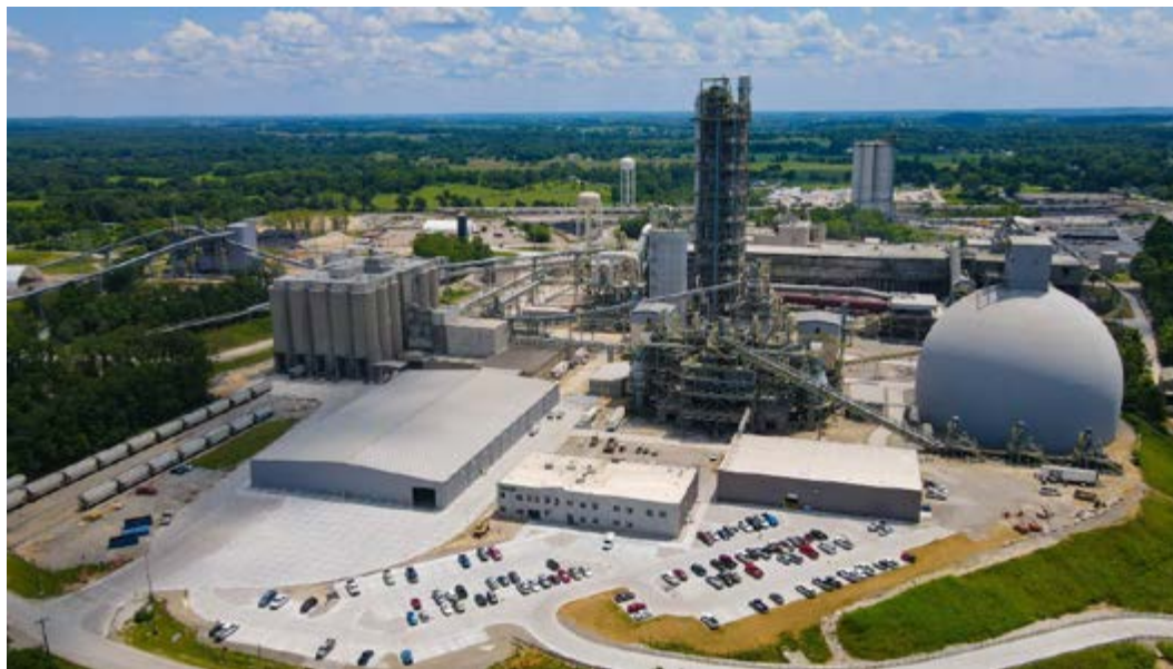
Figure 1: Heidelberg Materials' newly modernized Mitchell cement plant, the site for this FEED study.
