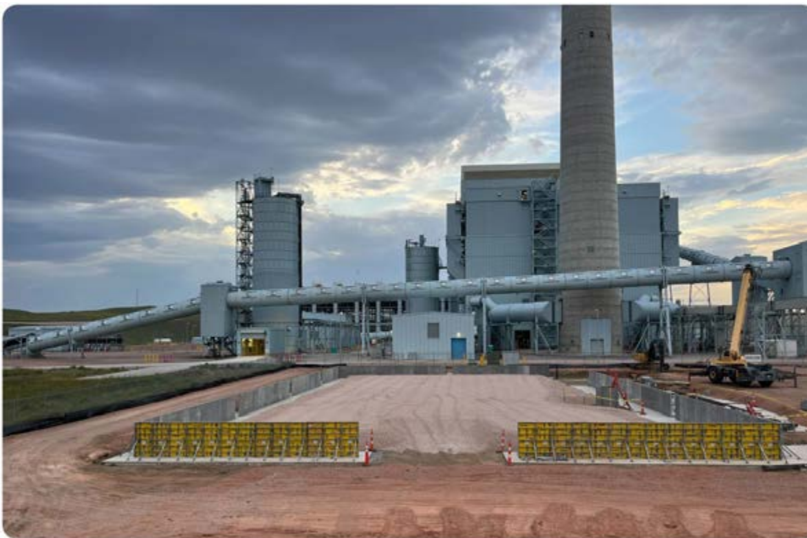
Figure 4: Preparation for equipment installation.
