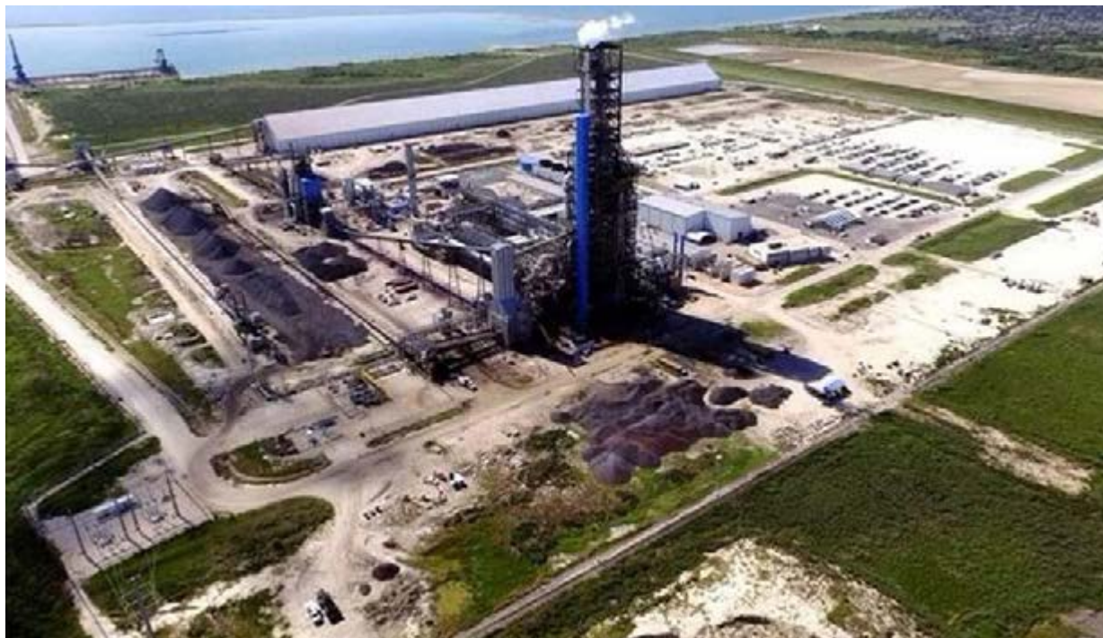
Figure 1: ArcelorMittal Texas HBI Facility in Portland, Texas.
