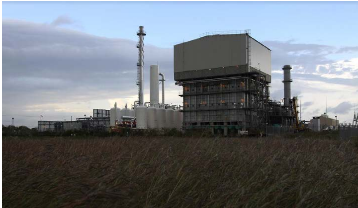
Figure 1: Air Liquide steam methane reformer at the La Porte, Texas, host site on the Gulf Coast.
