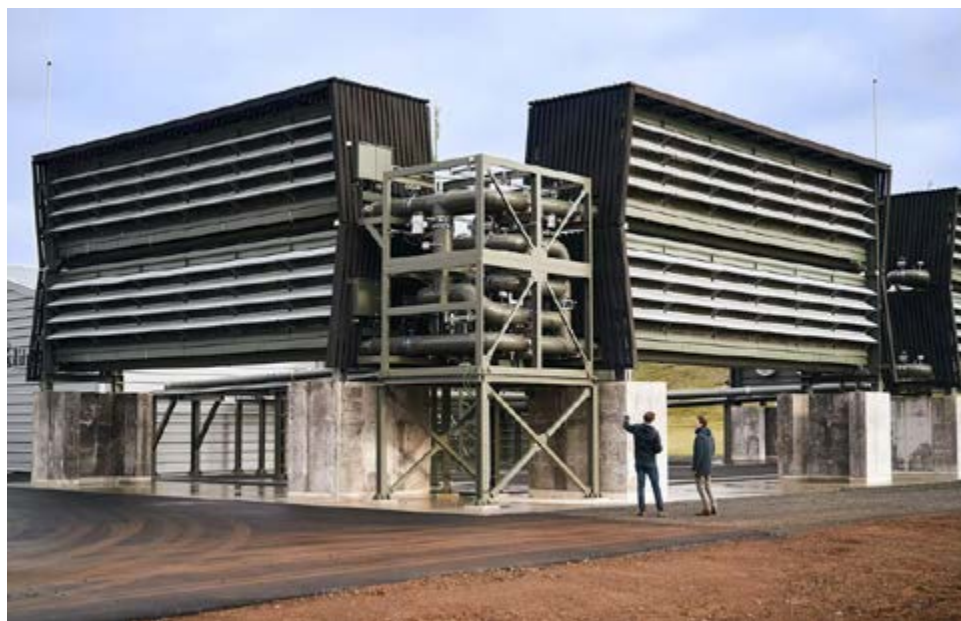
Figure 2: Climeworks' Orca plant, the world's largest direct air capture and storage plant, commissioned in Iceland in September 2021, with a capture capacity of up to 4,000 t CO2 /year.
