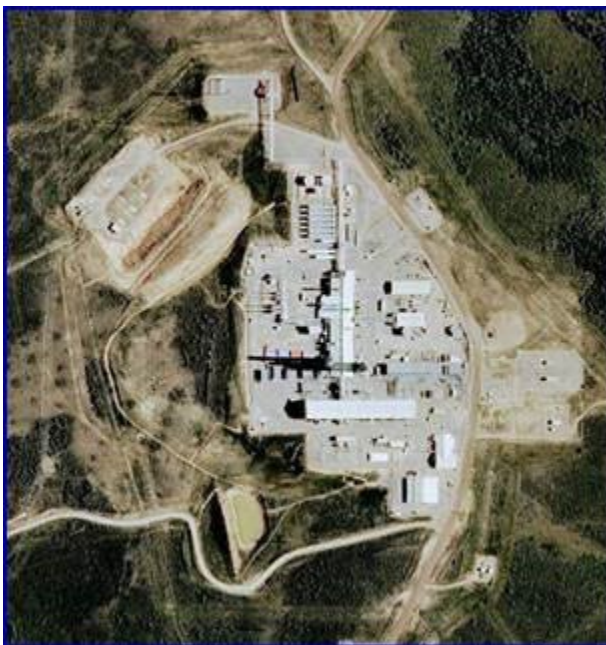
Figure 1: Proposed brownfield site for clean hydrogen plant in Evanston, Wyoming.
