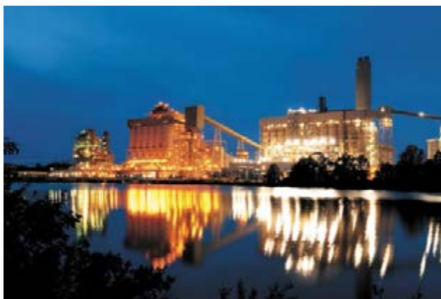
Figure 1: Cleco Power's Madison Unit 3 power plant.
