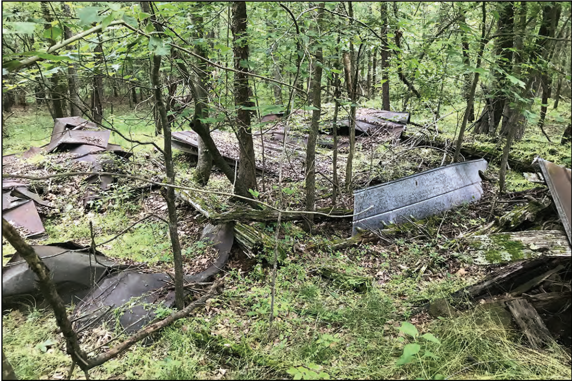
PLATE 6: Second Structure at Site 44PY0398
