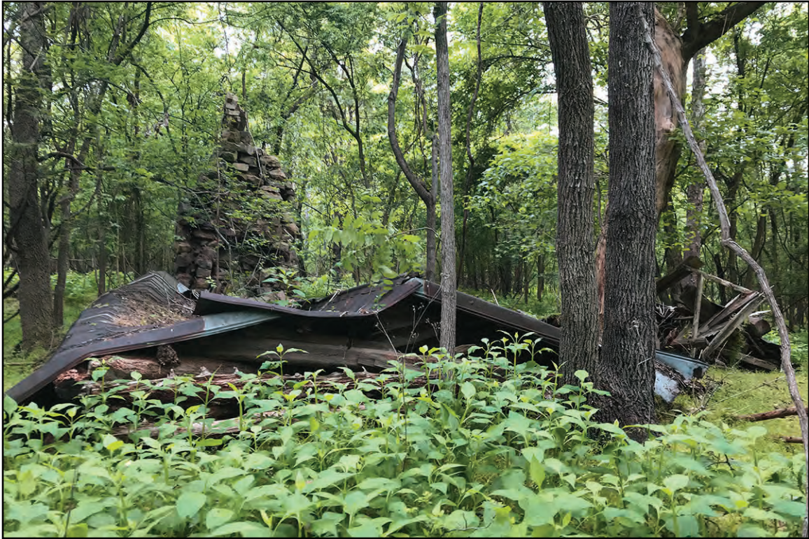
PLATE 4: Collapsed Cabin at Site 44PY0398, Facing Northwest
