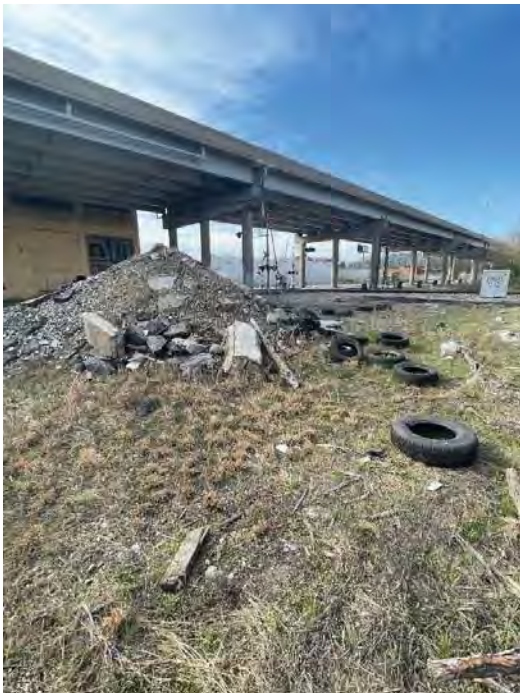
View of one of the many debris piles, containing tires and concrete, located on the southern side of the proposed project site.
