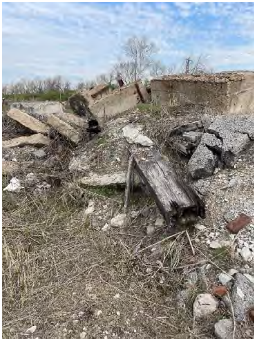
View of one of the several debris piles, containing concrete, asphalt, gravel, and rebar, located near the center of the proposed project site.
