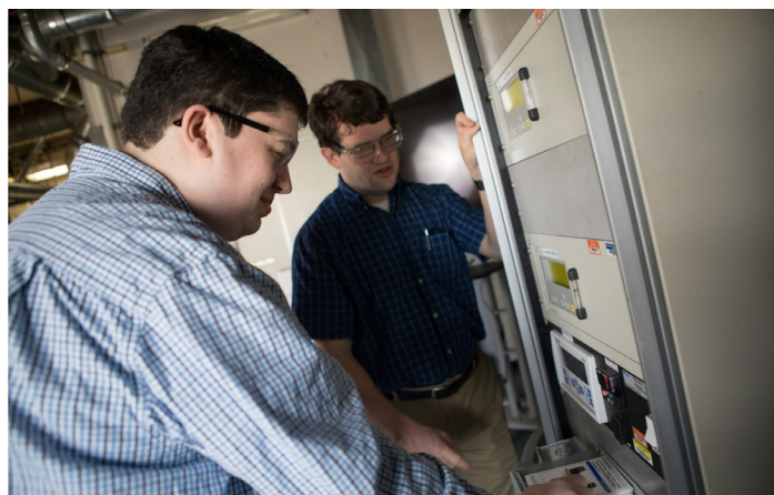
Figure 2. Researchers inspecting instrumentation measuring the outlet gas composition of the single fluid bed reactor.
