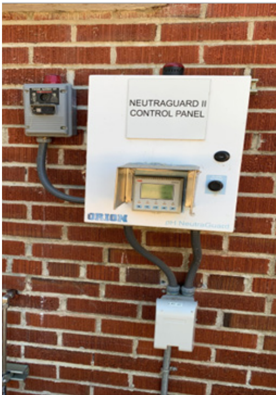
3.1.6.2a: Elementary neutralization system.
