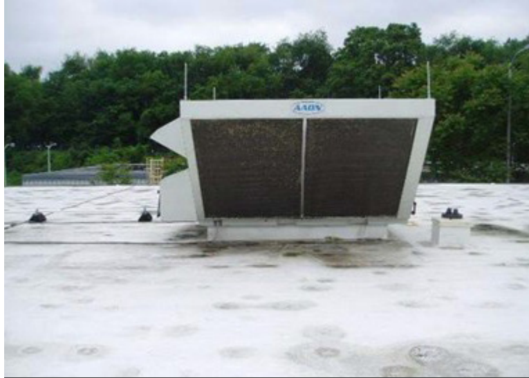
Photo 3.2.6.3: Pittsburgh air conditioner condensate.
