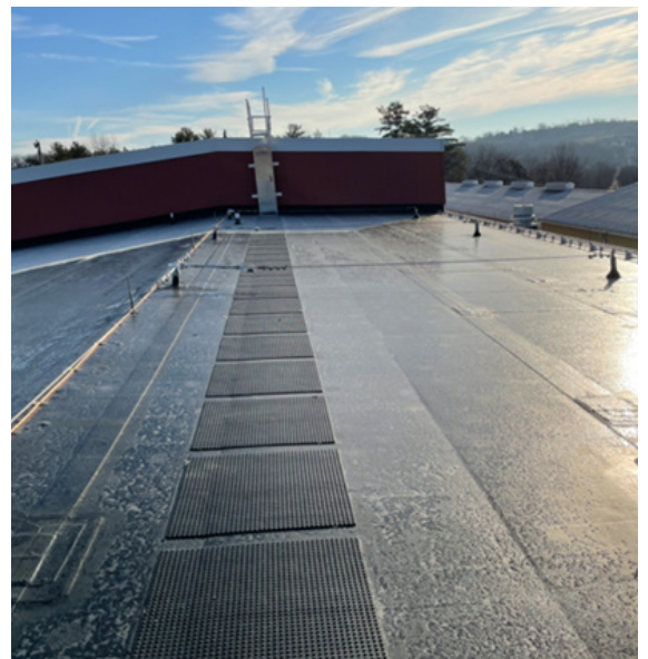
Photo 3.2.2m: B-167 — new roof with fall protection and lighting protection system.
