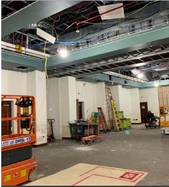
Photo 3.2.2c: B-922 conference center renovation – room 106.
