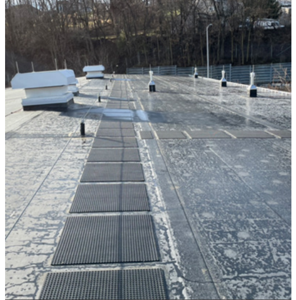
Photo 3.2.2k: B-901 — new roof with fall protection and lighting protection system.
