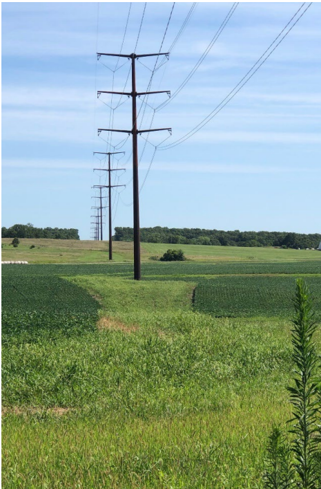
TYPICAL DOUBLE CIRCUIT 245 KV TANGENT STEEL STRUCTURE LINE POST FRAMING
