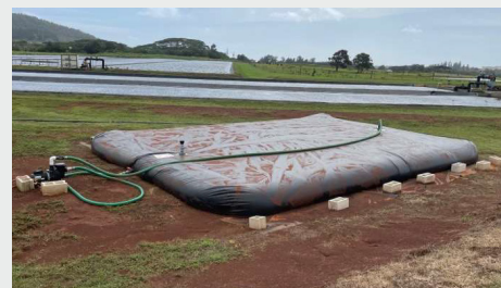
Carbonated Media Bladder Tank
