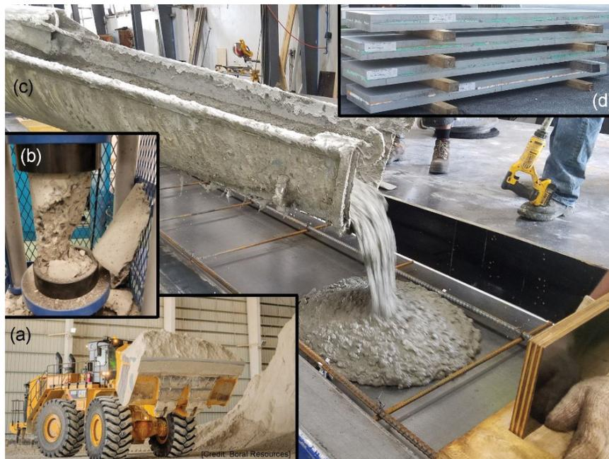
Development of a high-volume fly ash implementation framework for precast concrete construction will encompass (a) participation from a coal-fueled power generation facility and fly ash distributor, (b) cutting-edge concrete materials science research, and (c) fabrication and experimental testing of (d) full-scale precast components.
