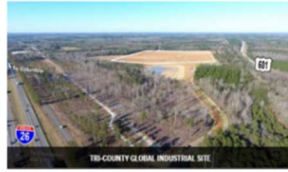
Tri- County Global Industrial Site
