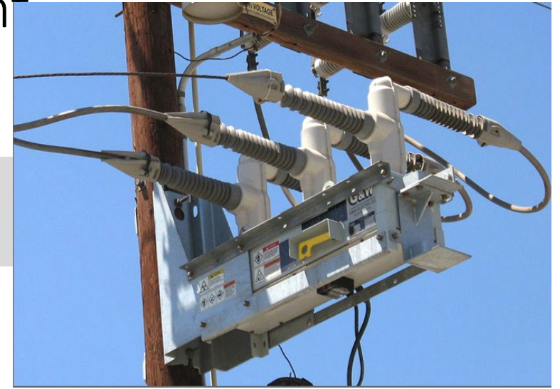
Example of an Autorecloser Device Proposed : Empire already operates multiple autoreclosers but seeks to expand the scope vi a focused 5-year sprint to bring a step change in reliability.
