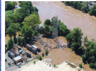
Pencoyd Flooding during Hurricane Ida
