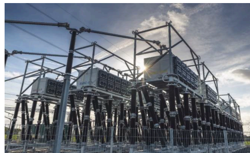
Figure 4. SmartValve installations at National Grid Electric Transmission Substation in England.
