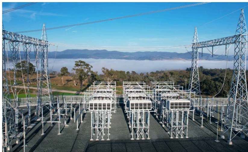
Figure 1. SmartValve installations at Transgrid substation in Australia.
