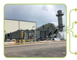
Primary heater included a hot section fabricated using IN 740H.
