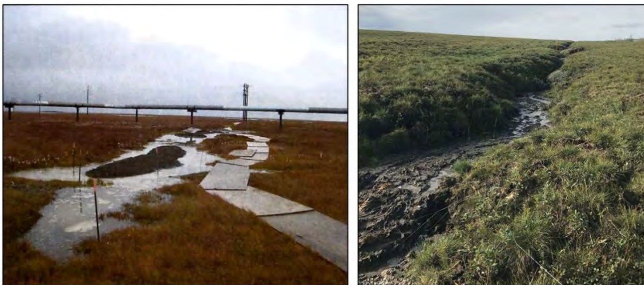
Figure 1. Ponding in wetland tundra along a utilities trench with mounded overburden to compensate for subsidence (left). Advanced subsidence and vertical erosion due to trenching and subsequent thaw of ice-rich permafrost on an incline (right). Both examples underwent several restoration attempts prior to photograph dates.
