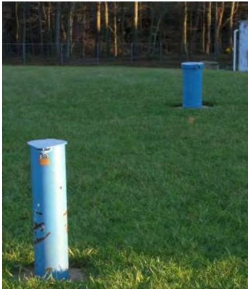
Photo 6.0: Morgantown monitoring wells.
