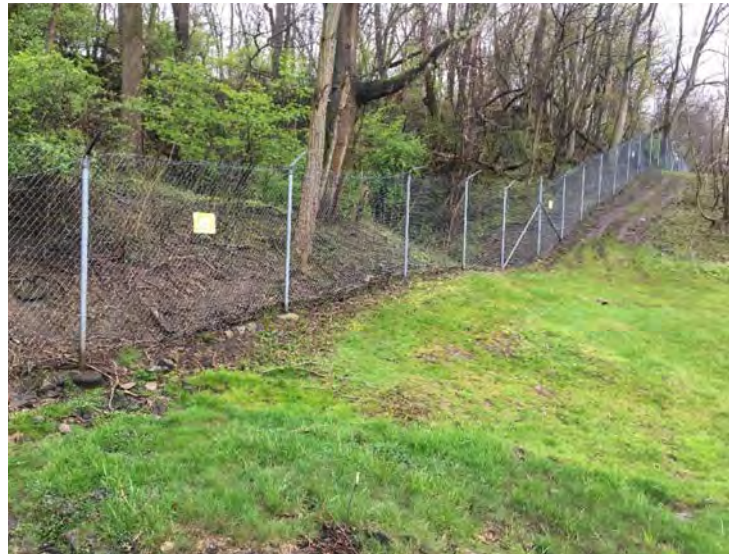
Photo 3.3.2.8b: 900/920 plateau perimeter fence replacement.
