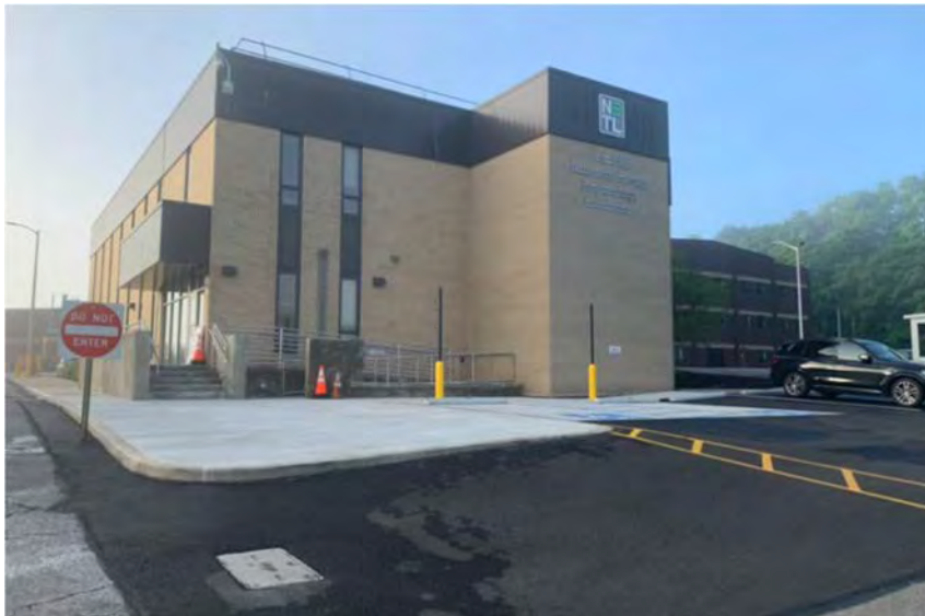
Photo 3.3.2.11a: B-920 renovation – additional parking and ADA ramp.
