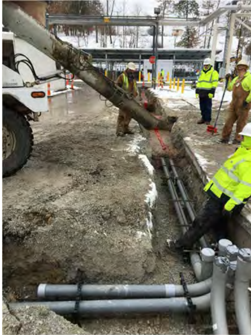
Photo 3.3.2.12b: R&D plateau electrical conduit installation.
