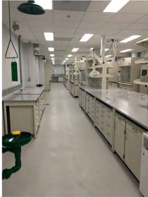
Photo 3.3.2.1b: B-94 second floor – after renovation.
