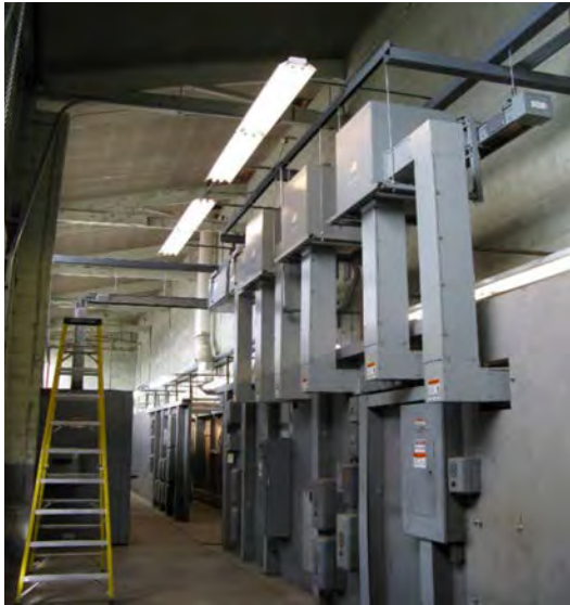
Photo 3.2.2.1: B-28 electrical vault upgrades design.
