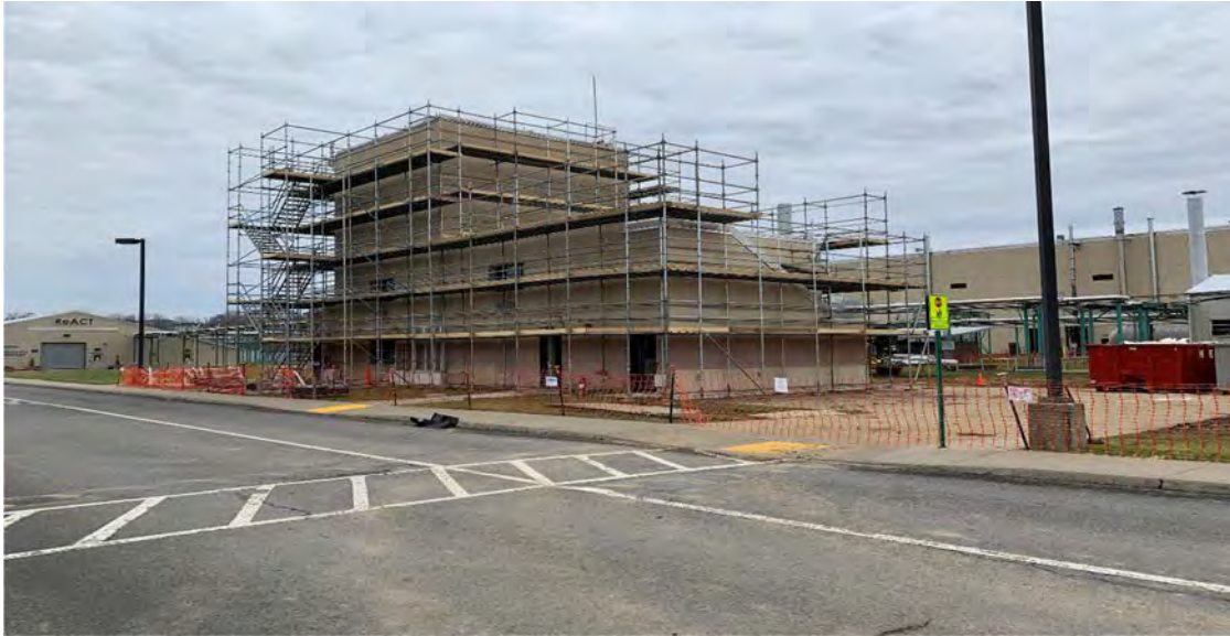
Photo 3.5.2.3a: B-7, previous security building; demolition in process.
