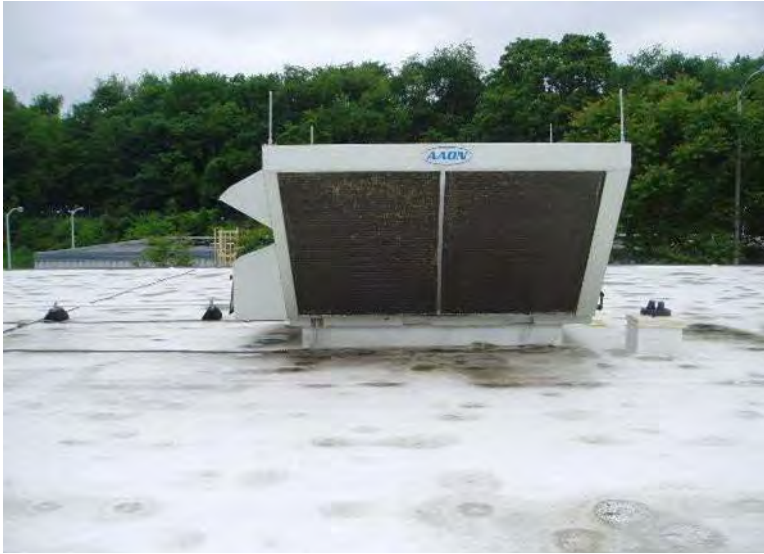
Photo 3.3.6.3: Pittsburgh air conditioner condensate.
