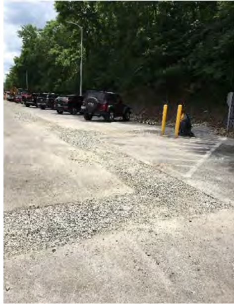
Photo 3.3.2.2b: 920 plateau area – near end of construction.
