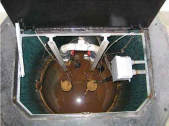
Photo 3.5.6.1a: Morgantown parking lot oil-water separator.
