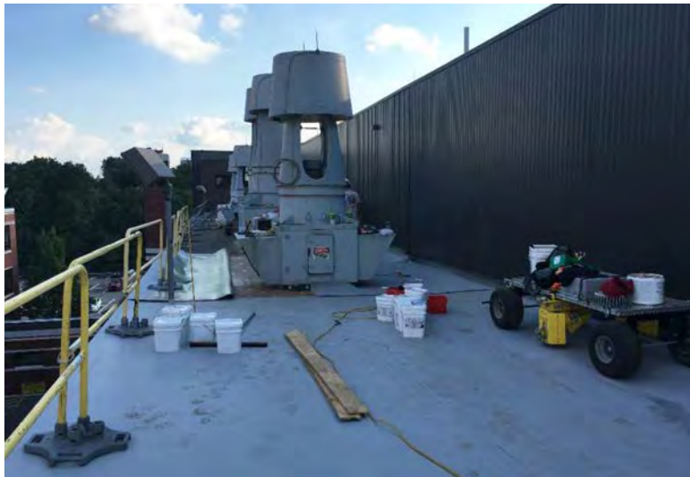
Photo 3.3.2.7: B-84 roof replacement – new roof in foreground, old roof in background.
