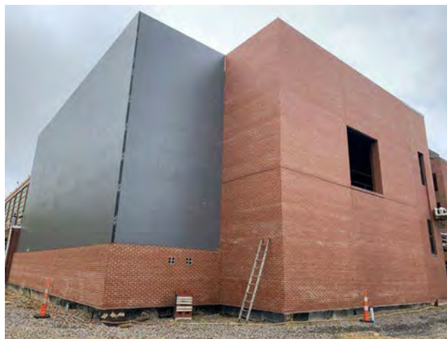
Photo 3.3.2.4: B-83 CDAML – building addition.
