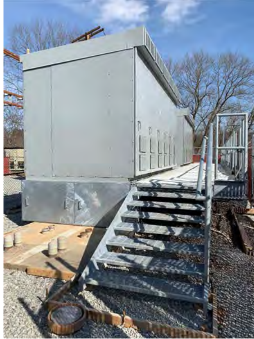
Photo 3.3.2.5: Substation 6 – new switchgear.
