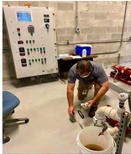
Photo 3.5.6.1d: Weekly pH monitoring at the Morgantown pH control facility (water leaving the clarifier).
