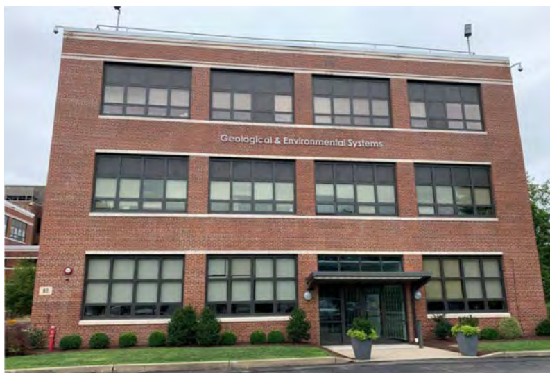
Photo 3.3.2.9: B-83 brick repointing – B-83 South after brick repointing.
