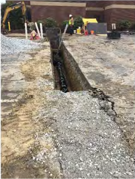
Photo 3.3.2.2a: 920 plateau area – before/during construction.
