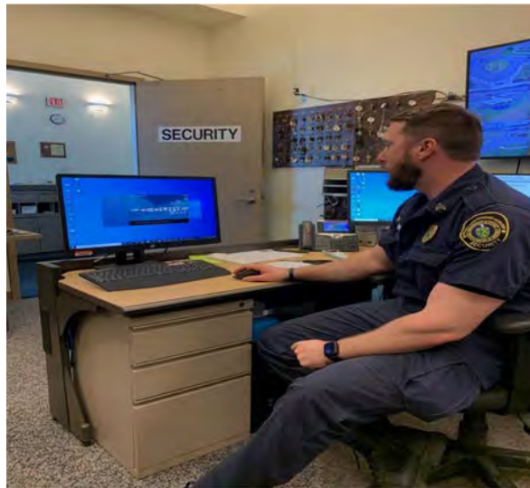
Photo 3.5.2.2b: Access control workstation.
