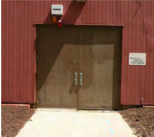
Photo 3.3.2.10a: Door replacement – B-922-door 7S before replacement.
