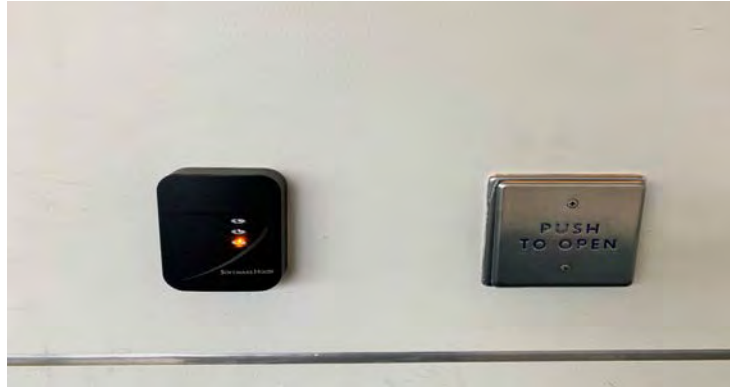
Photo 3.5.2.2a, Access control card reader.
