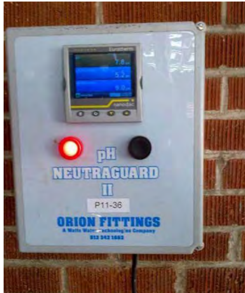
Photo 3.2.6.2: Elementary neutralization system.
