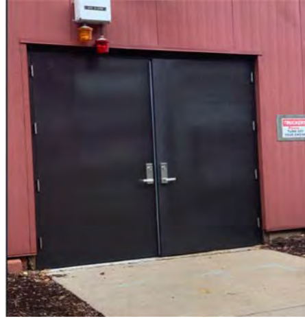
Photo 3.3.2.10b: Door replacement – B-922-door 7S after replacement.
