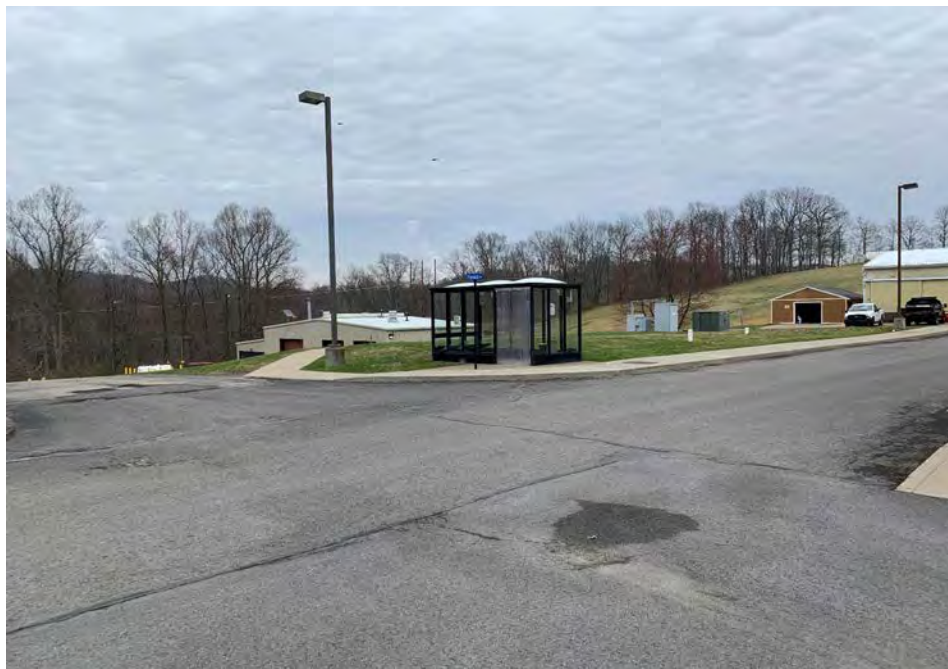
Photo 3.5.2.3b: Site of future Morgantown security building.
