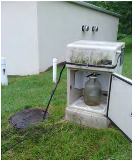
Photo 3.5.6.1c: Morgantown wastewater permit sampling point.
