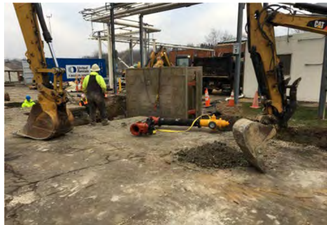
Photo 3.3.2.12a: R&D plateau fire line replacement.
