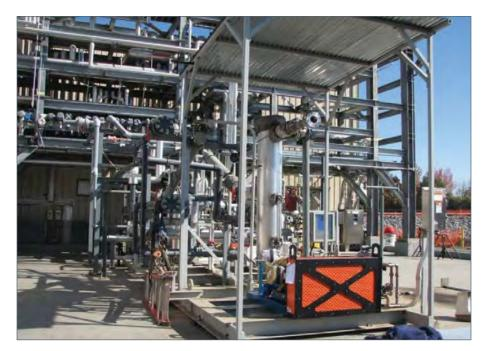
Figure 4: Membrane skid used for 1-TPD bench-scale slipstream testing at NCCC.
