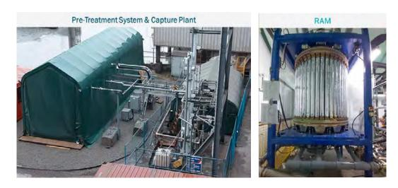
Figure 3: CO<sub>2</sub>MENT field Unit (1 TPD) at a Lafarge cement plant in Richmond BC showing the pre-treatment system and capture plant (left) and the RAM showing the beds (right).
