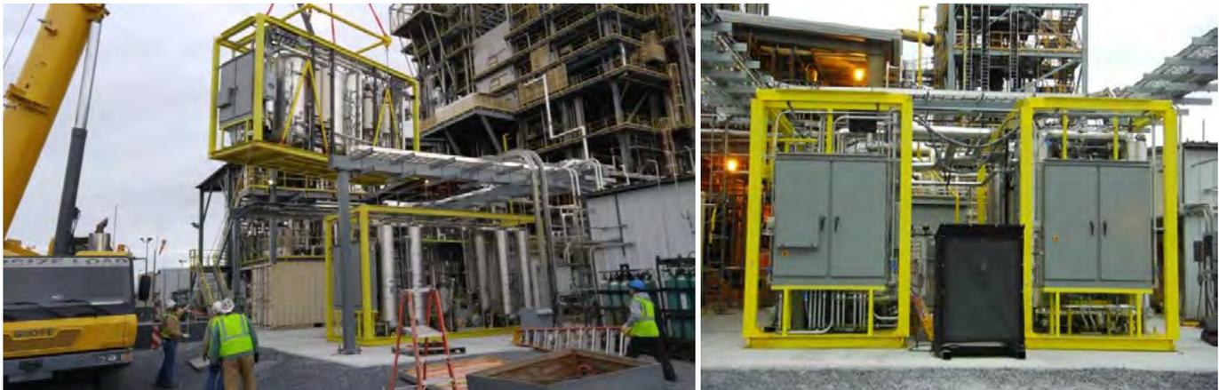
Figure 4: TDA’s 0.1-MWe pilot unit installed in the test pad at the NCCC (Wilsonville, Alabama).
