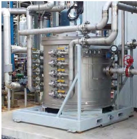
Figure 6: Prototype plate-and-frame module during testing at NCCC.
