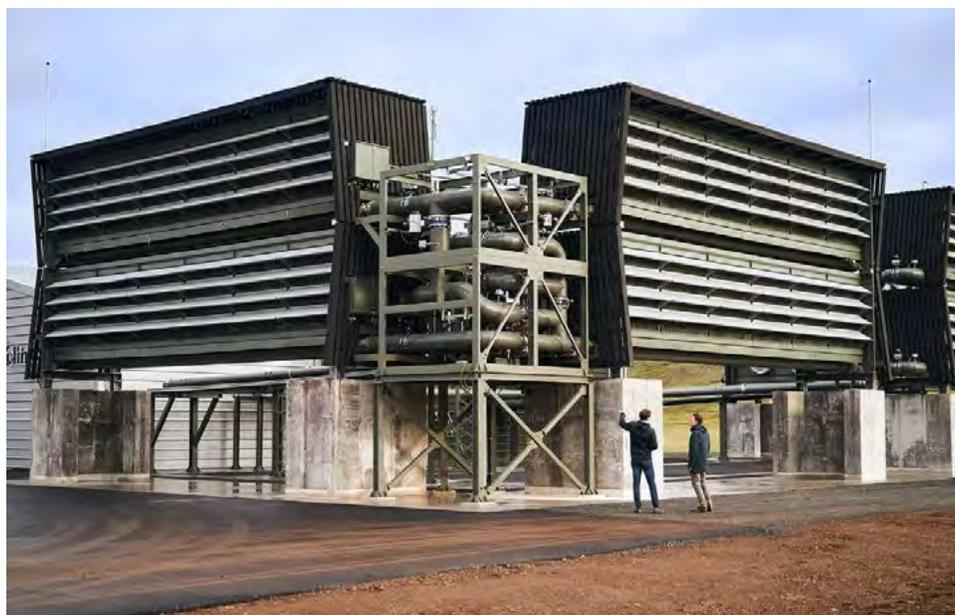
Figure 2: Climeworks' Orca plant, the world's largest direct air capture and storage plant, commissioned in Iceland in September 2021, with a capture capacity of up to 4,000 tCO<sub>2</sub>/year.
