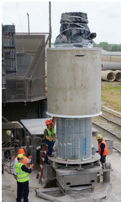
H 2 Storage Tank.
