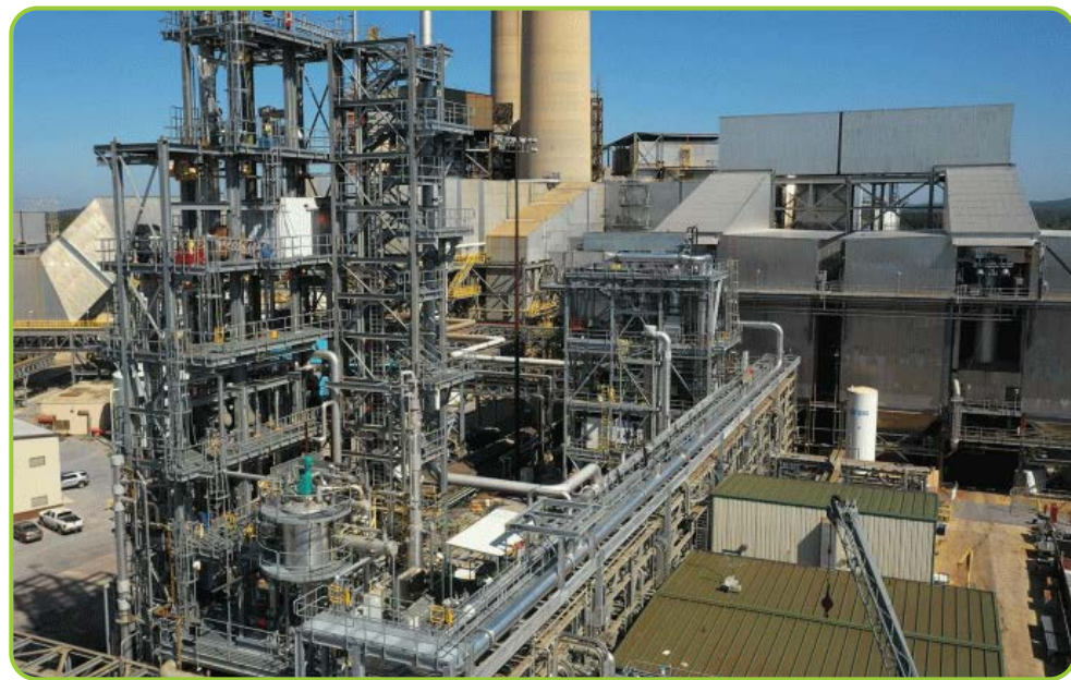
NCCC at Alabama Power's Plant Gaston in Wilsonville, Alabama
