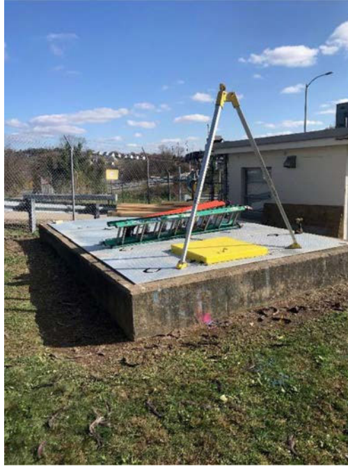
Photo 3.3.2.7: B-911 Water Pit Cover – Under Construction.
