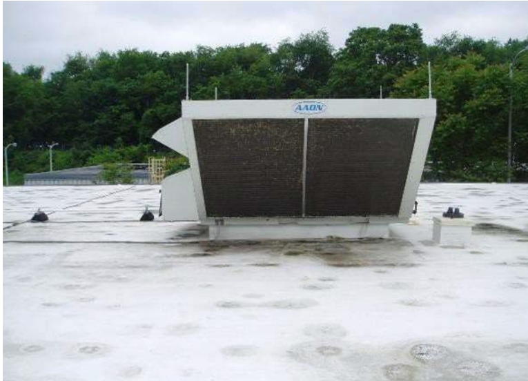
Photo 3.3.6.1: Pittsburgh Air Conditioner Condensate.
