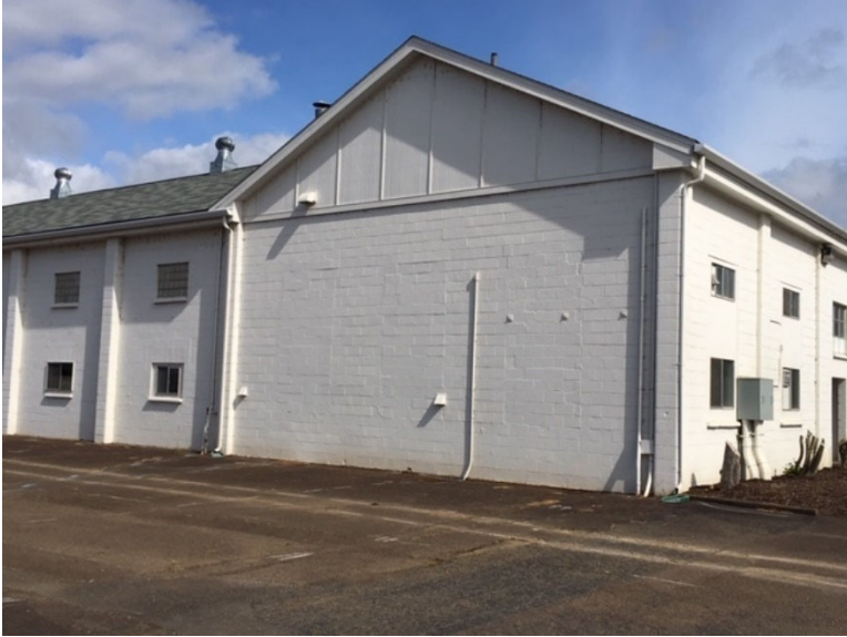
Photo 3.2.2.6: B-17 East Wing Renovation Design
