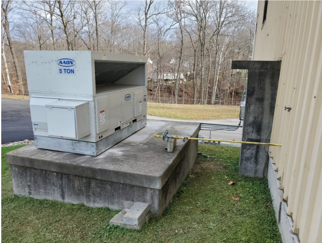
Photo 3.5.2.7: Building 17 Laboratory HVAC Replacement
