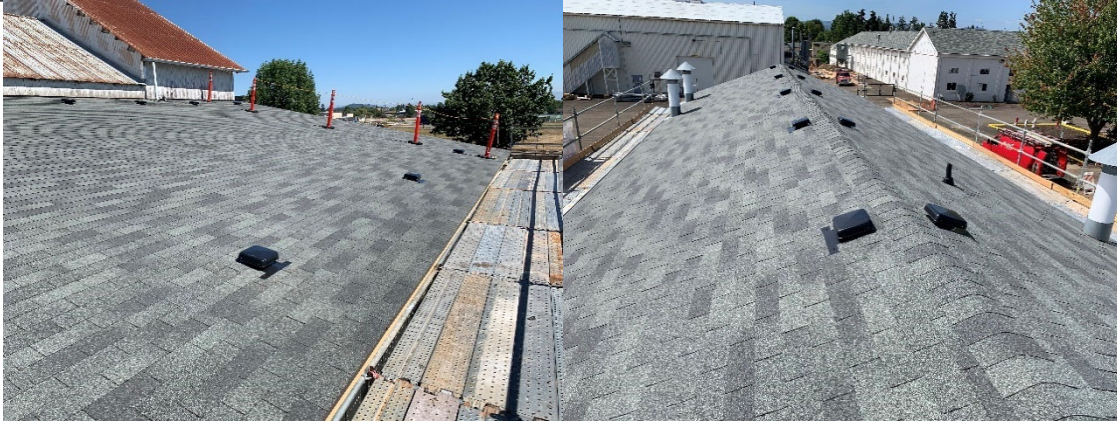
Photo 3.2.2.4: B-24 & B-35 Asphalt Roof Replacements
