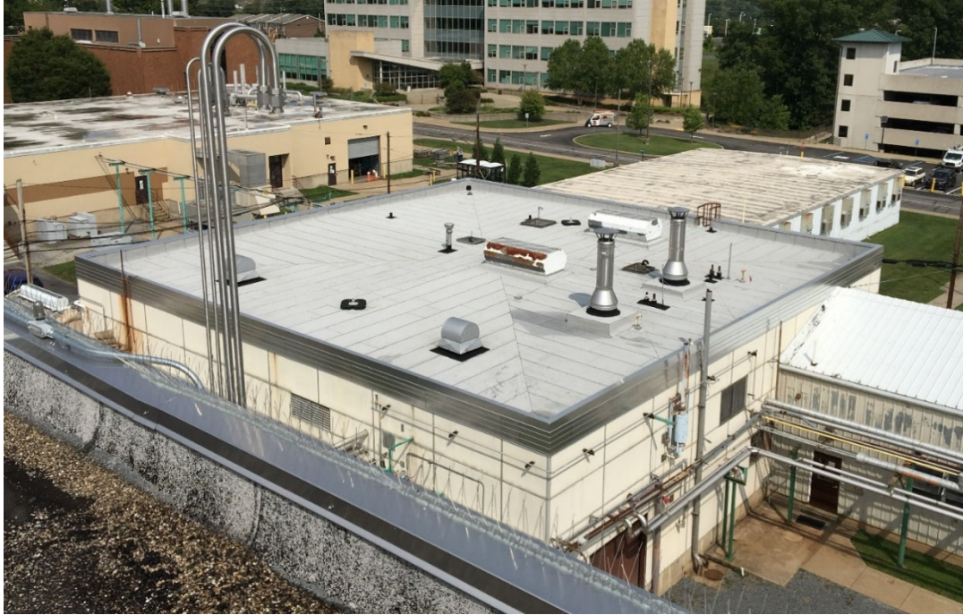
Photo 3.5.2.2: Building 5 Roof Replacement
