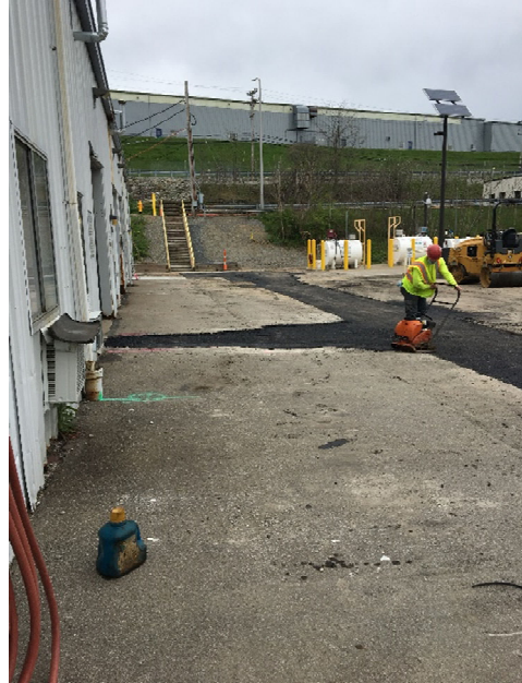
Photo 3.3.2.2b: 900 Plateau Area – Near End of Construction.
