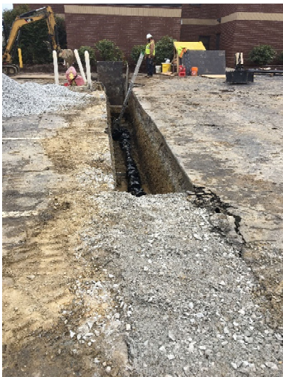
Photo 3.3.2.3a: 920 Plateau Area Before/During Construction.
