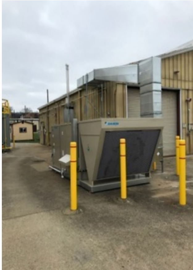
Photo 3.5.2.6: New Building 13 HVAC Unit
