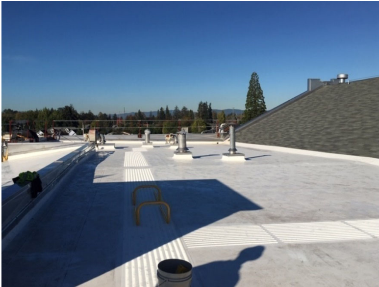
Photo 3.2.2.5: B-23 Roof Replacement
