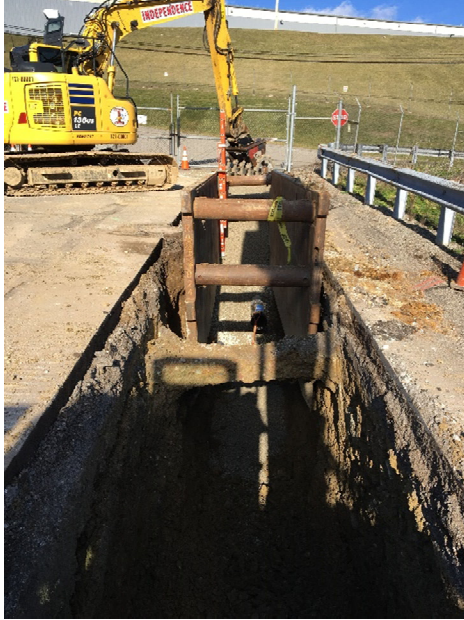
Photo 3.3.2.2a: 900 Plateau Area – Before/During Construction.
