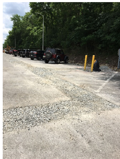
Photo 3.3.2.3b: 920 Plateau Area Near End of Construction.
