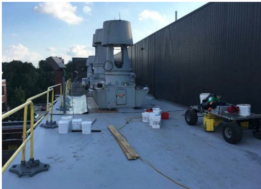
Photo 3.3.2.6: B-84 Roof Replacement – New roof in foreground, old roof in background.
