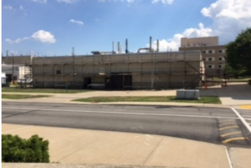
Photo 3.5.2.5: Building 3 During EIFS Renovation
