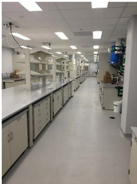
Photo 3.3.2.1c: B-94 Second Floor – After Renovation.
