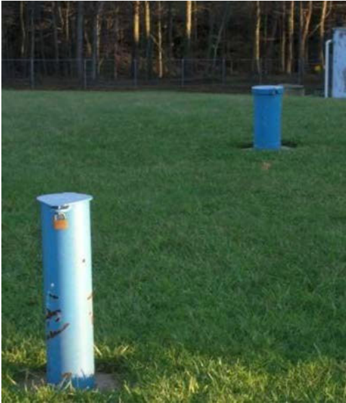
Photo 5.0: Morgantown Monitoring Wells.
