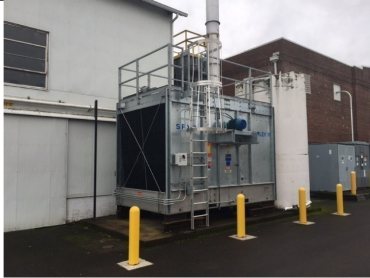
Photo 3.2.2.2: B-23/24 Cooling Tower Replacement
