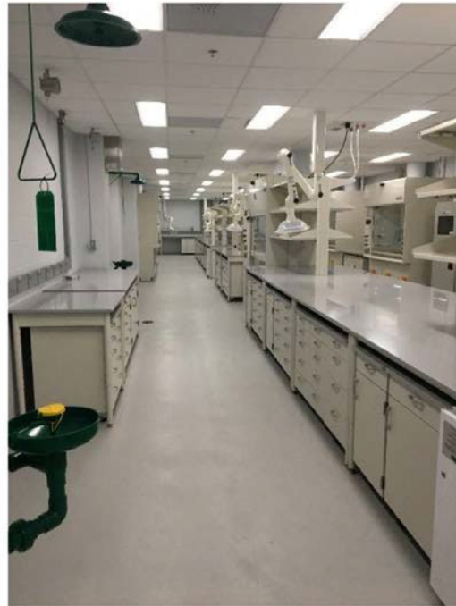
Photo 3.3.2.1b: B-94 Second Floor – After Renovation.
