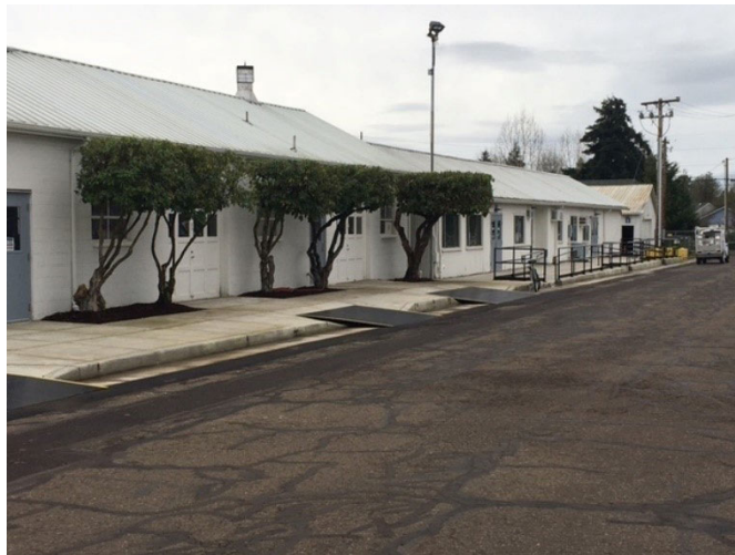
Photo 3.2.2.3: B-7 through B-11 Sidewalk & Drainage Upgrades
