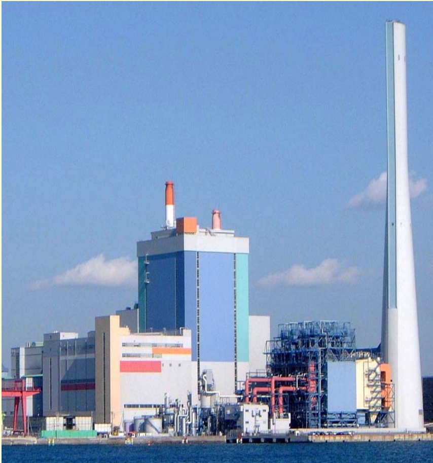
Photo of Shin-Isogo Unit. 1
