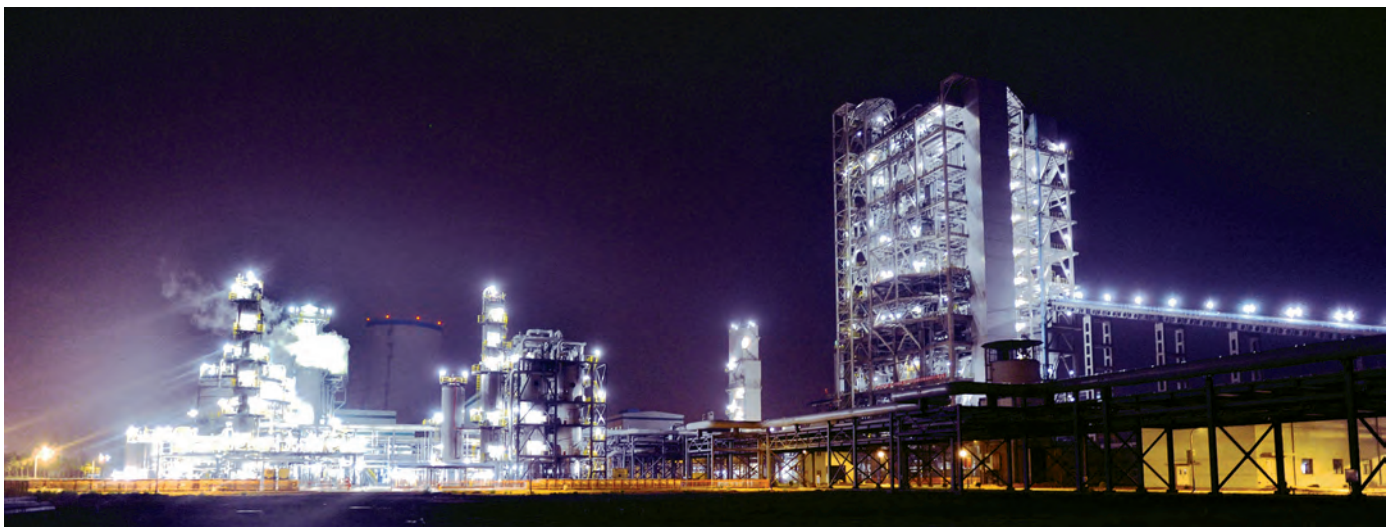
A 250-MW capacity IGCC power station was designed, constructed, and operated under Phase I of the GreenGen Plan.
