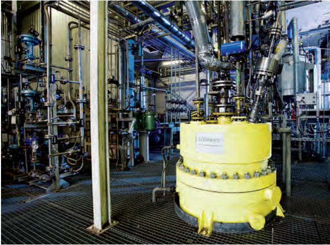
FIGURE 2. Siemens Fuel Gasification Test Center, 5-MW th gasifier
