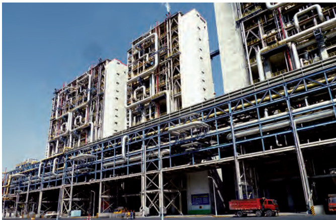
Shenhua Ningxia Coal Group’s coal-to-polypropylene project, Ningxia Province, PRC
