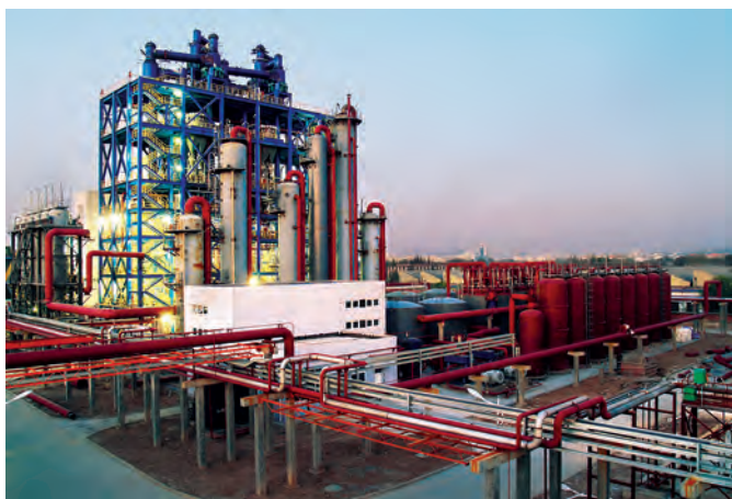
SES’ Zao Zhuang New Gas Company Joint Venture Plant that produces methanol from coal—Shandong Province, China (SES ~98% ownership)
