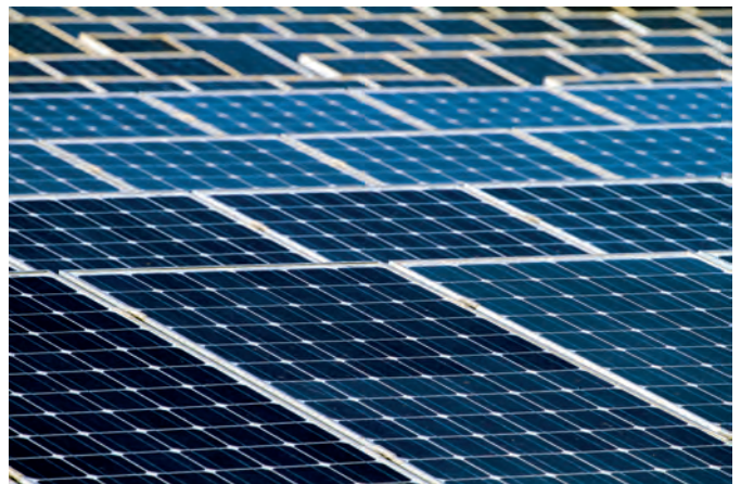
Large and small solar power installations also have a role in Modi's energy plan.
