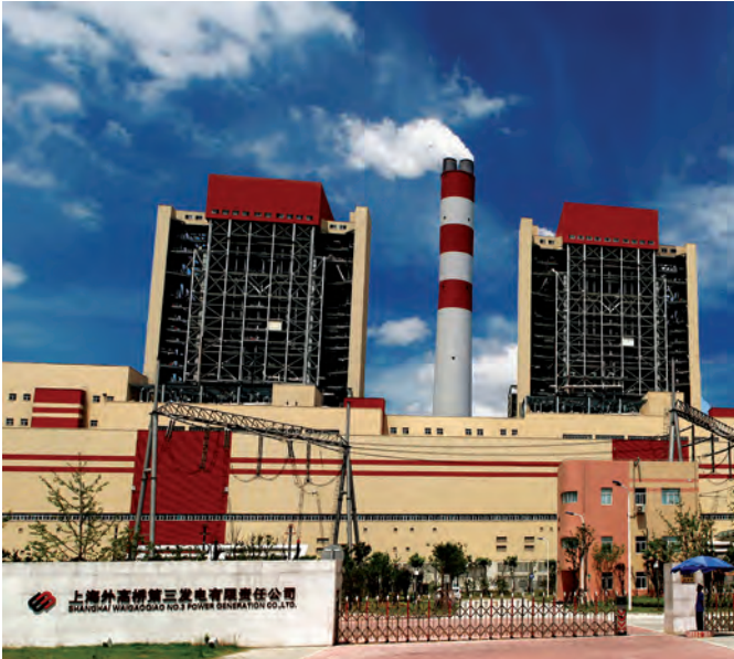
The Shanghai Waigaoqiao No. 3 power plant is one of the many high-efficiency power plants built in China in recent years.
