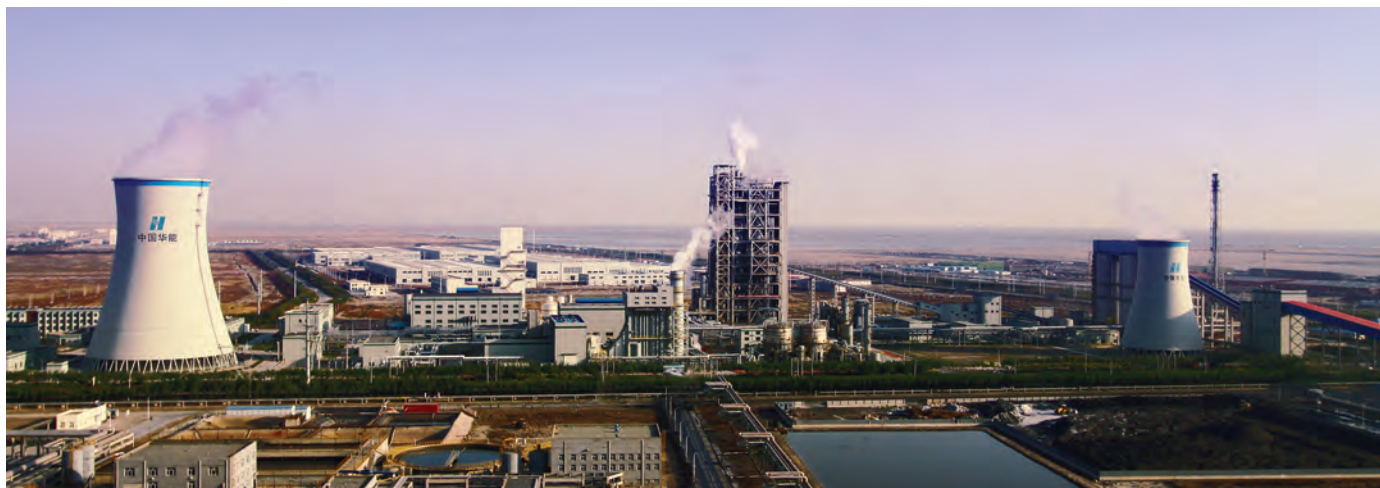
The full Phase I GreenGen IGCC facility is shown above.
