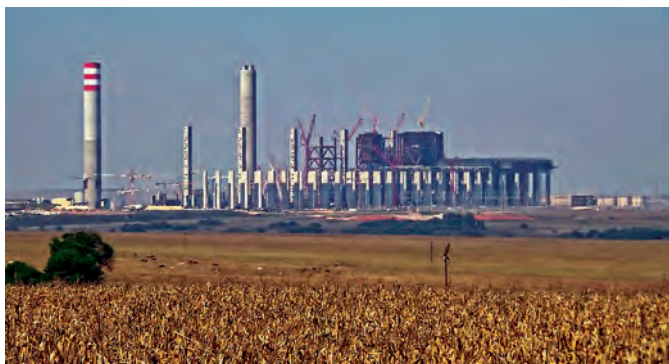
Eskom is working to increase the efficiency of its coal fleet. The under-construction Kusile power plant is shown above.
