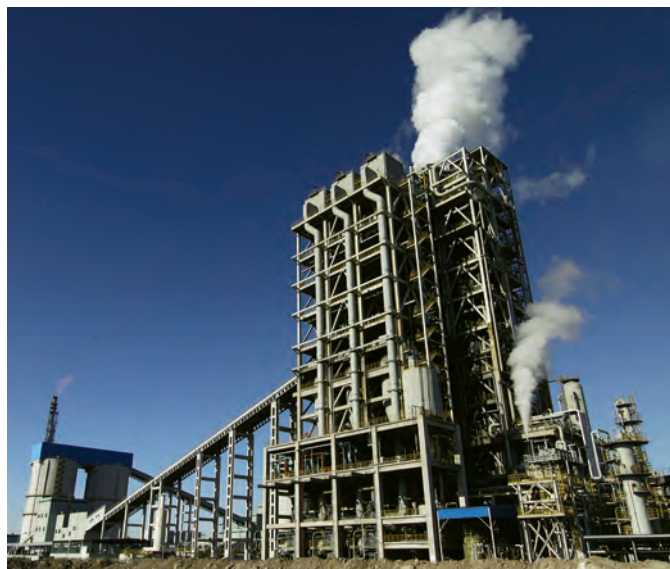
The Chinese-developed gasifier used in Phase I of GreenGen is shown above.
