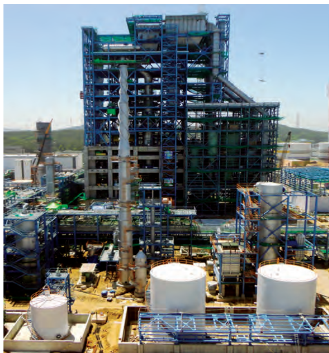
Gasification unit under construction at South Korean IGCC power plant (photo courtesy of Korea Western Power Co. Ltd)
