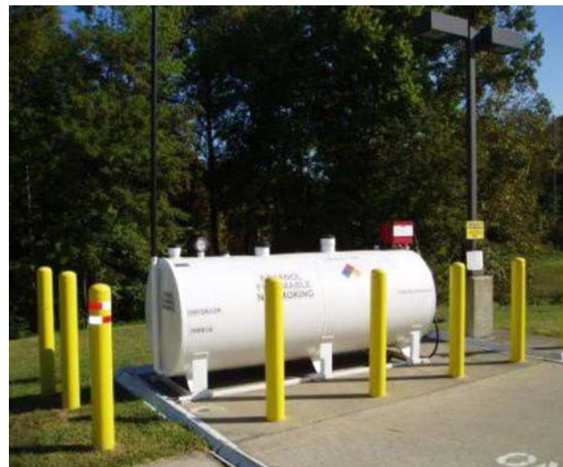
Photo 3.1.6.2.3: Ethanol Storage Tank.
