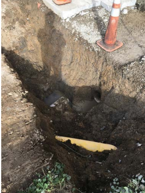
Photo 3.1.2.6: Main Sanitary Gravity Drain Line and the Building 19 South Line.
