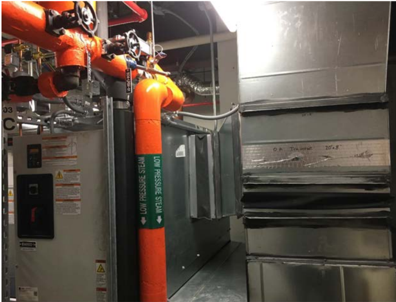
Photo 3.1.2.4: Building 4 HVAC Replacement.
