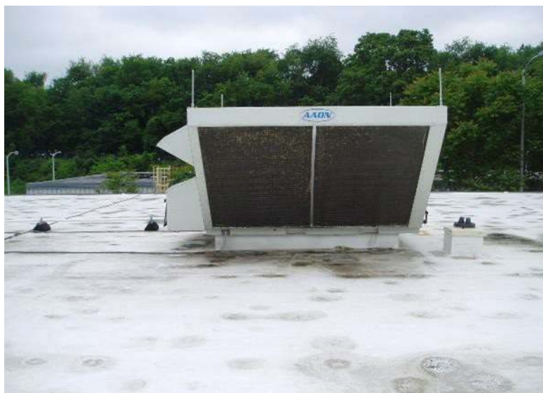
Photo 3.2.6.1: Pittsburgh Air Conditioner Condensate.
