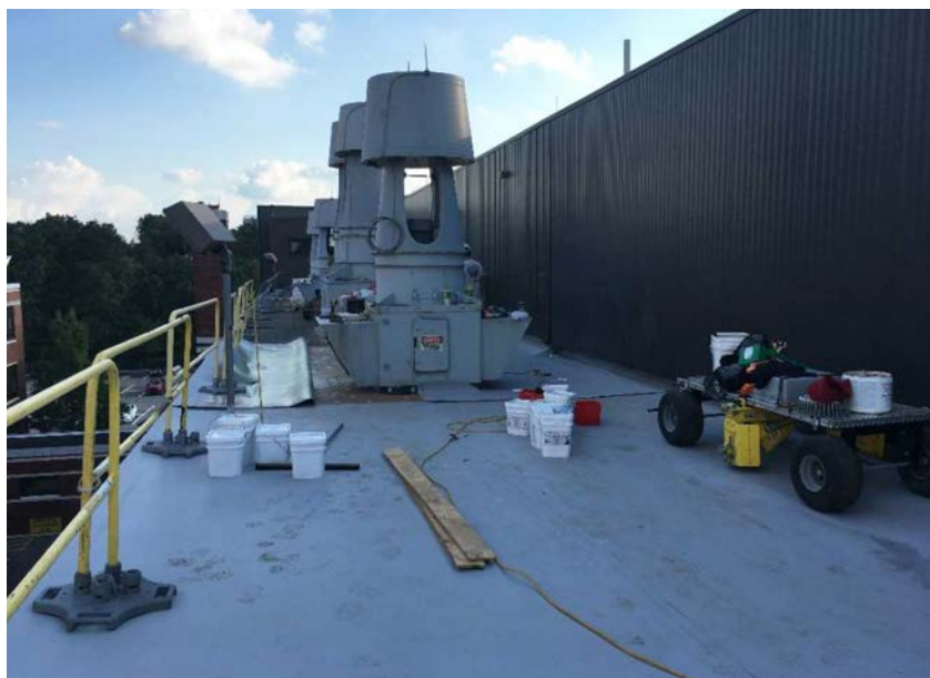
Photo 3.2.2.7: B-84 Roof Replacement – New roof in foreground, old roof in background.
