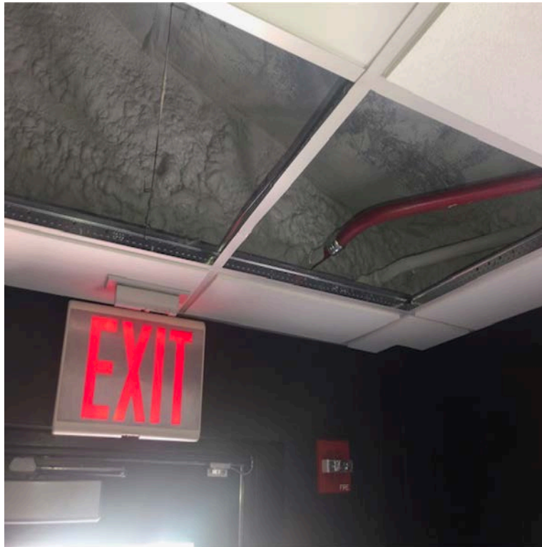
Photo 3.1.2.1: Control Room Insulation.
