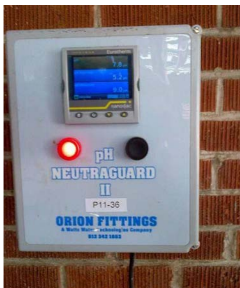
Photo 3.3.6.2: Elementary Neutralization System.
