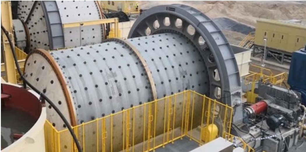
Figure 2-6 Typical Ball Mill Installation
