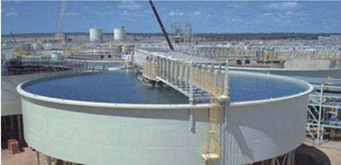
Figure 2-9 Typical Thickener Installation
