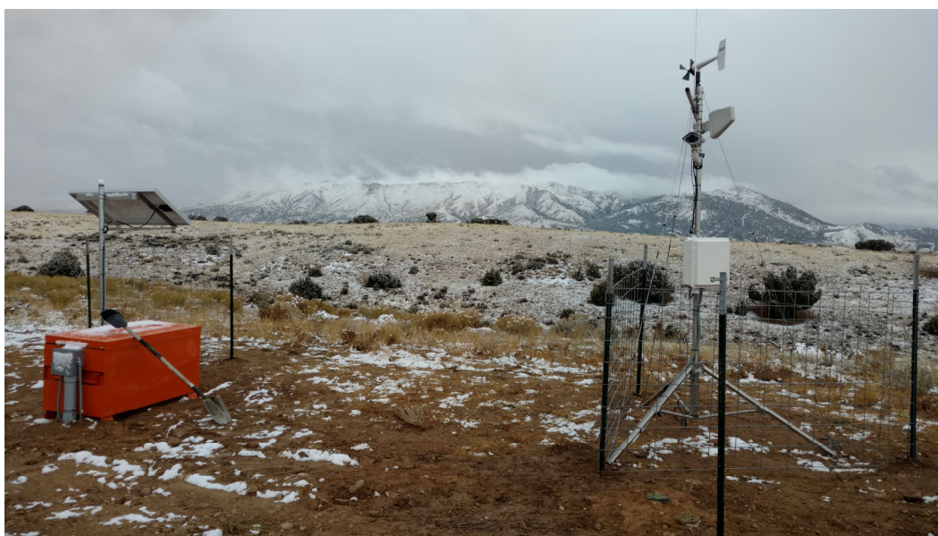
Figure G-2. Completed Meteorological Tripod Power/Control Box at Clay Basin Well
