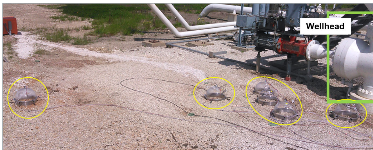
Figure 2-6. Longitudinal Flux Chamber Setup. The wellhead is outlined in green, flux chambers are circled in yellow.
