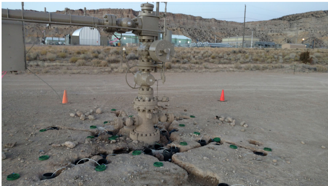
Figure G-1. In-ground Sensor and Sample Tubing Installation in Progress
