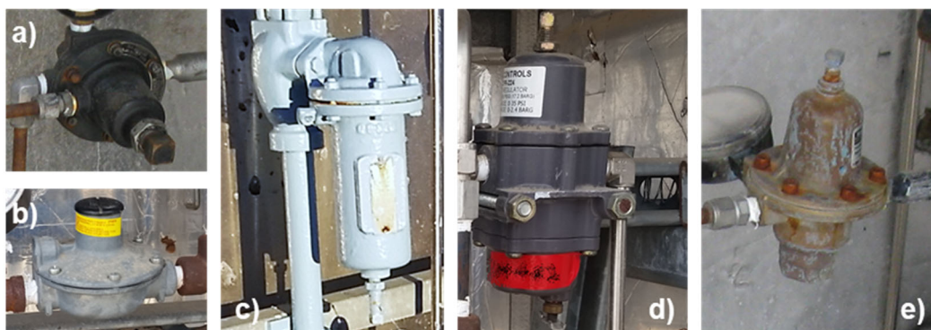
Figure B-7. Examples of Regulators on Underground Natural Gas Storage Wellheads
