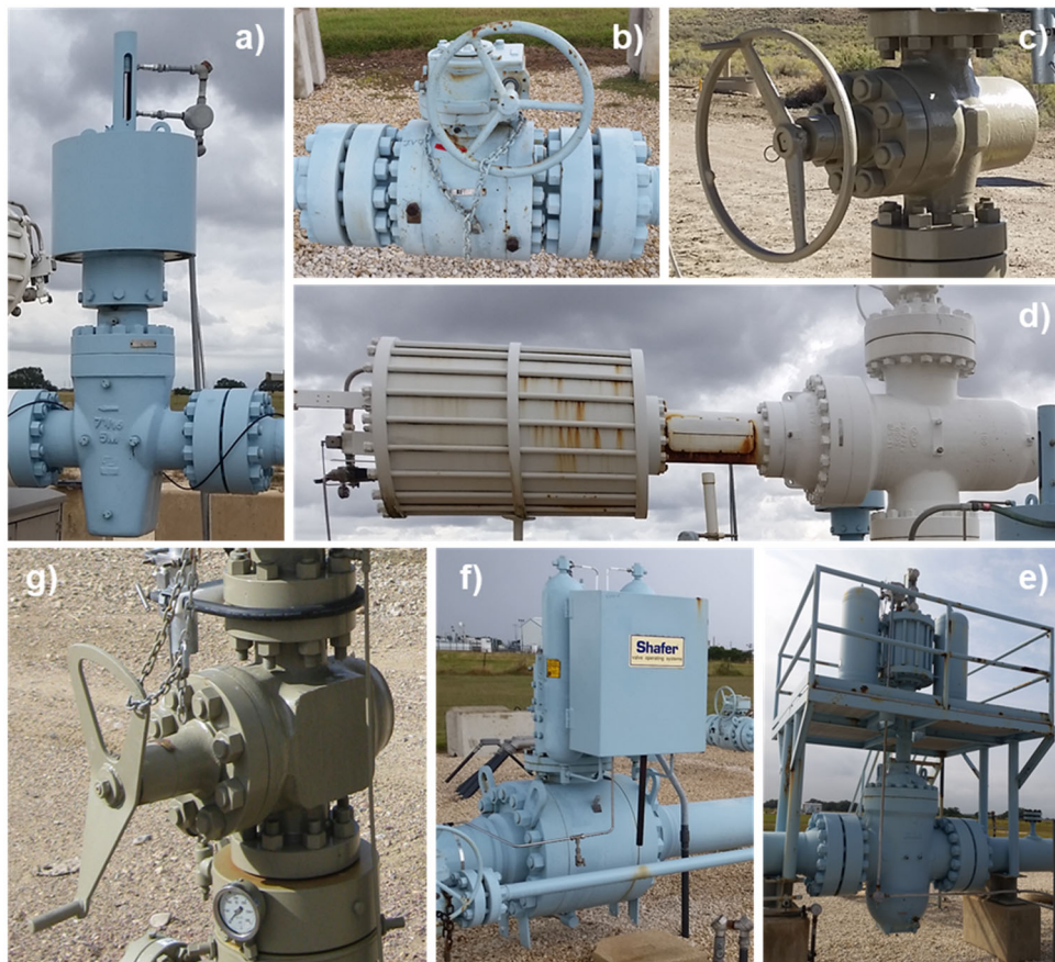
Figure B-3. Examples of Large Valves on Underground Natural Gas Storage Wellheads
