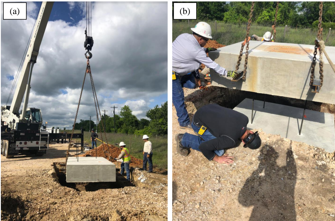
Figure 6. Field installation of surface orbital vibrator (SOV) steel reinforced modular concrete foundation. (a) Crane lowering bottom block into excavation; (b) Top and bottom SOV foundation blocks being assembled together.
