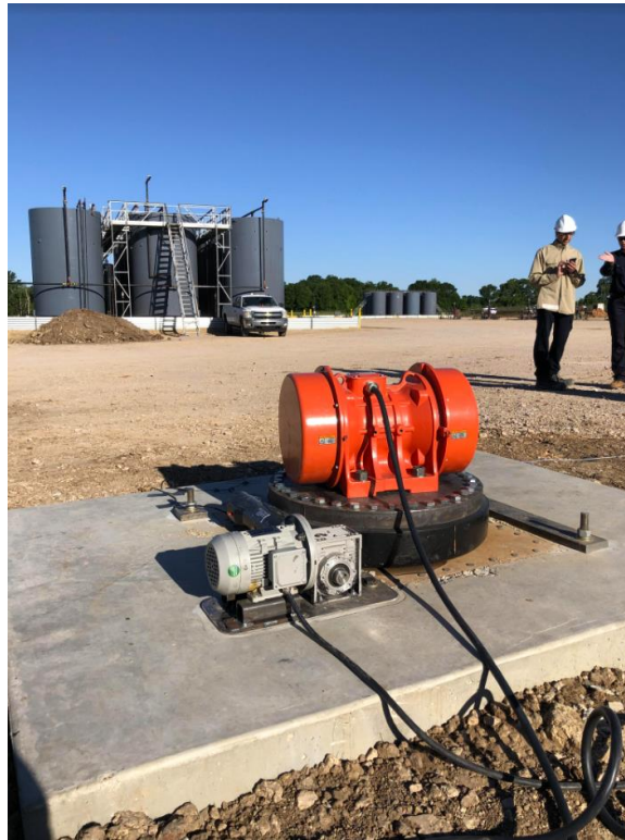
Figure 7. Completed Surface Orbital Vibrator (SOV) installation on Marjorie-Bartlett well pad.
