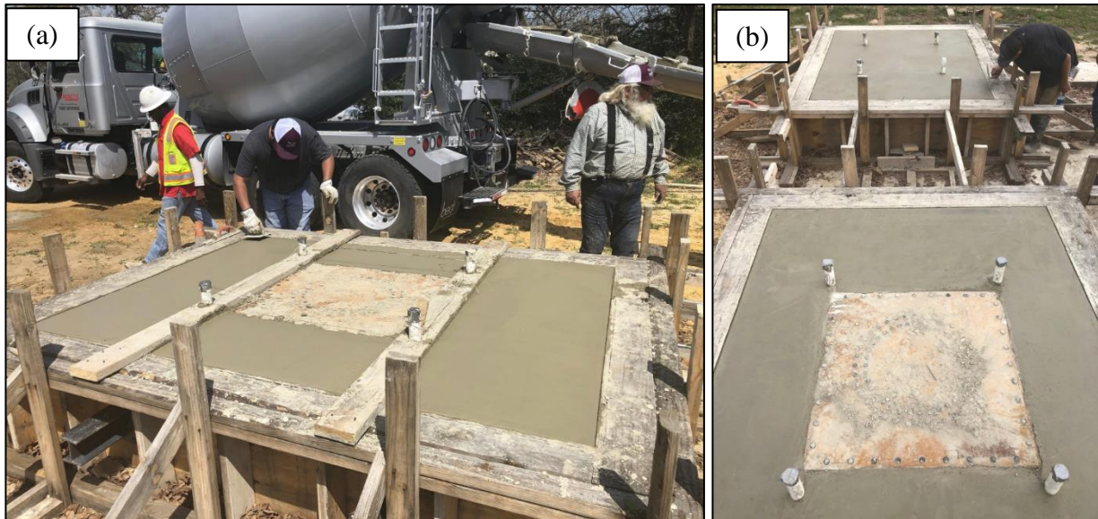
Figure 5. Completed surface orbital vibrator (SOV) steel reinforced modular concrete foundation. (a) Top foundation block with SOV mounting reinforcement; (b) Top and bottom SOV foundation blocks (to be assembled together to form complete SOV foundation).
