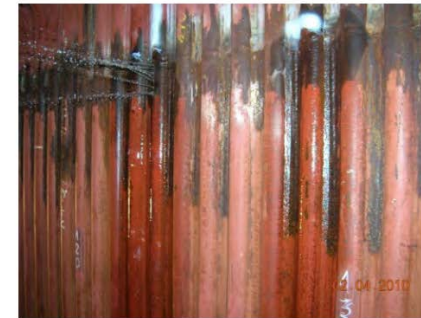
Cracks in longitudinal direction
