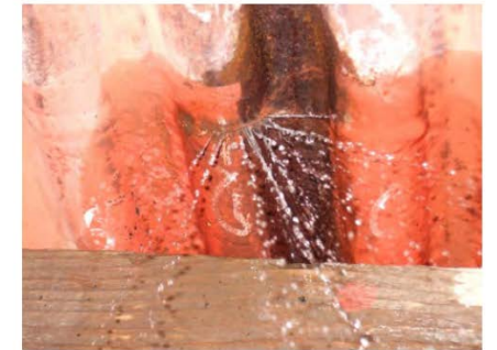
Cracks in transversal direction
