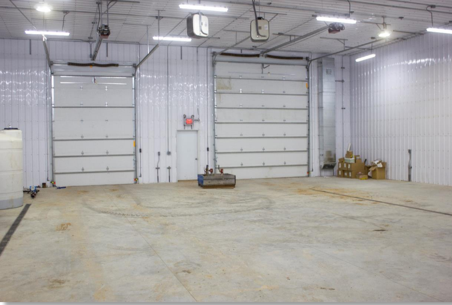
Demonstration Bay and Effluent Storage
