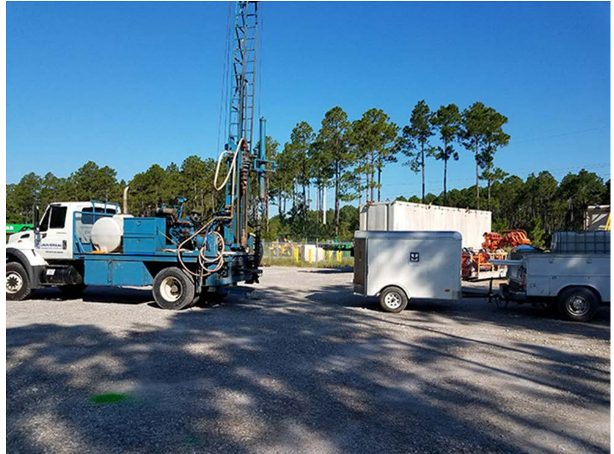
Monitoring well installation
