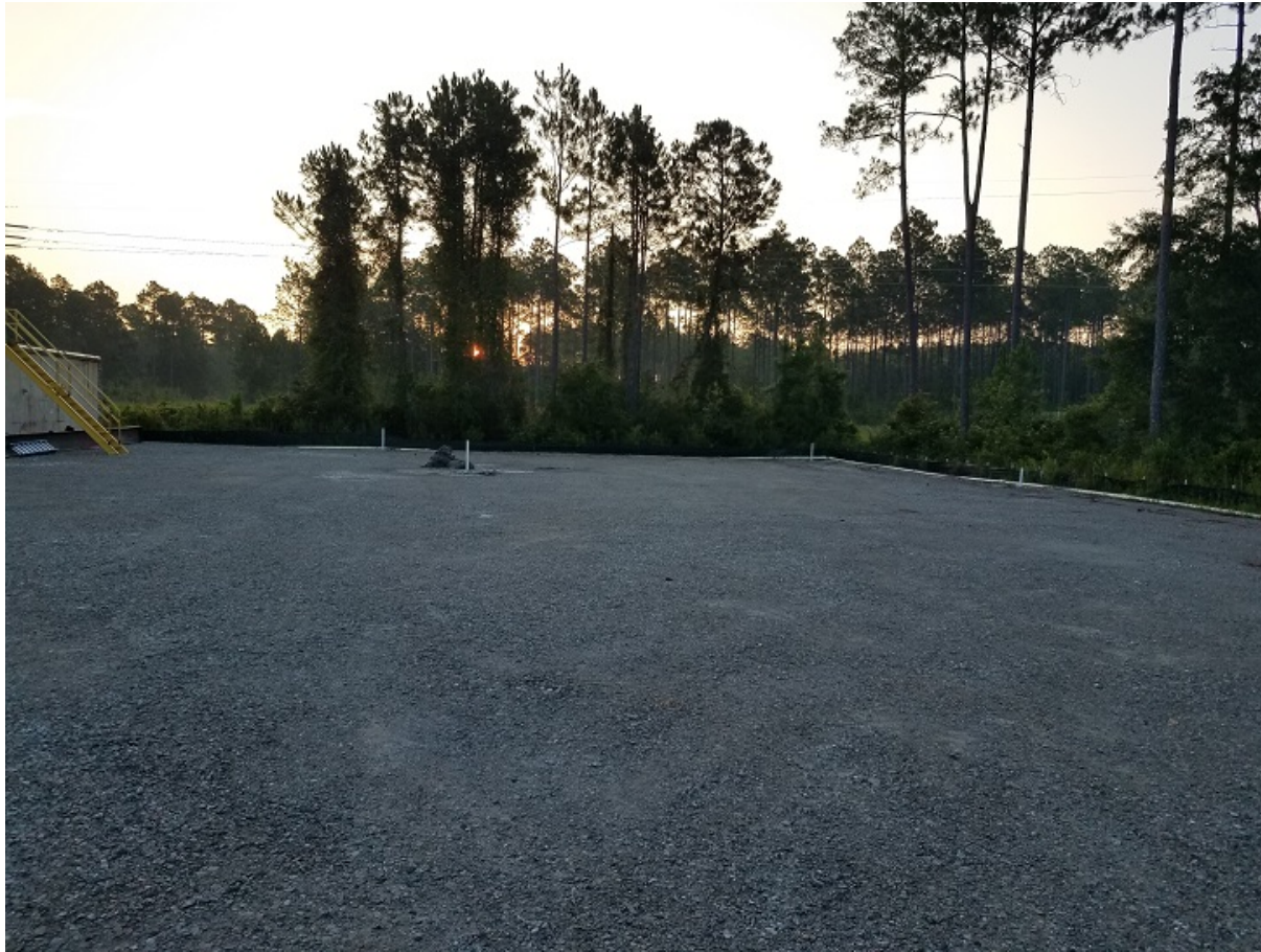
Drill pad installation
