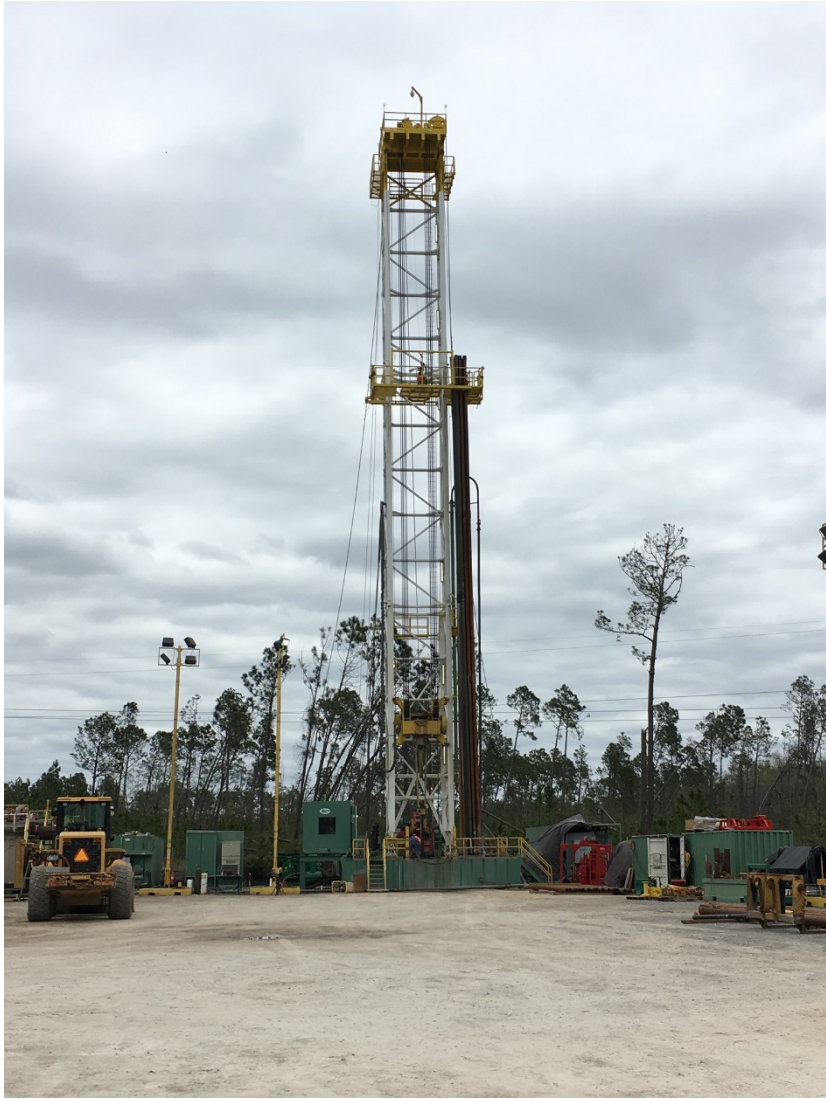
Electric rig drilling injection well TIW-2
