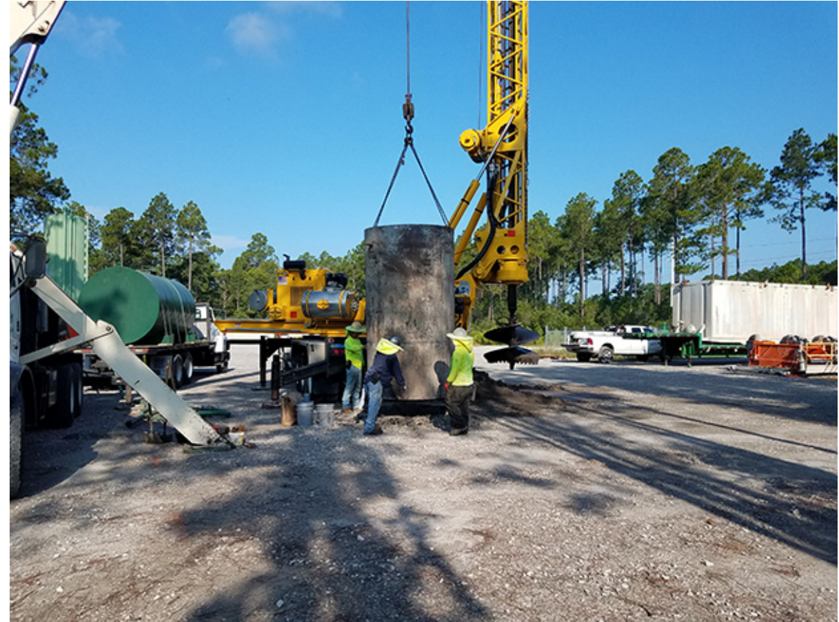
Installation of the 48-inch conductor casing
