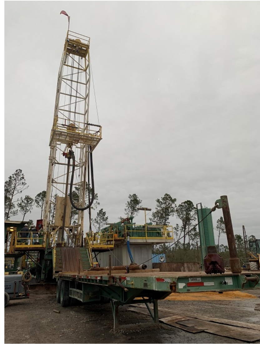
Diesel rig drilling observation well TEMW-A
