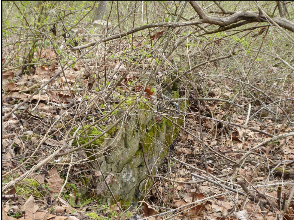
Figure 35: South foundation wall, facing southwest.
