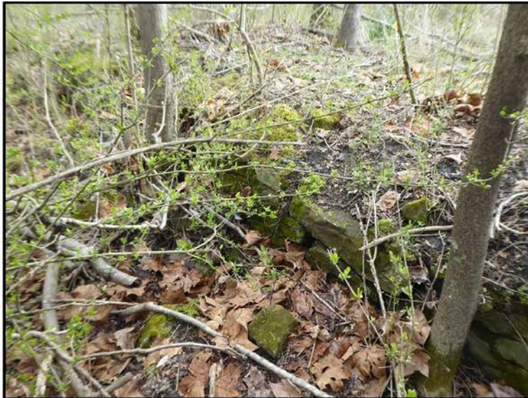
East foundation wall, facing north.
