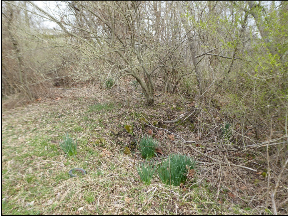
Figure 29: Site area facing southwest. Note south foundation wall in center of photograph.
