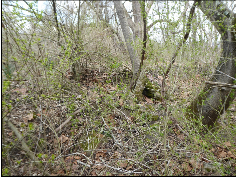
Figure 37: Foundation interior, facing west.
