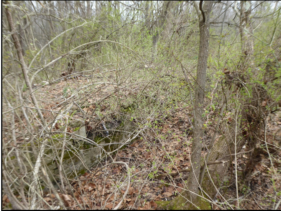
Figure 33: North foundation wall, facing northeast.
