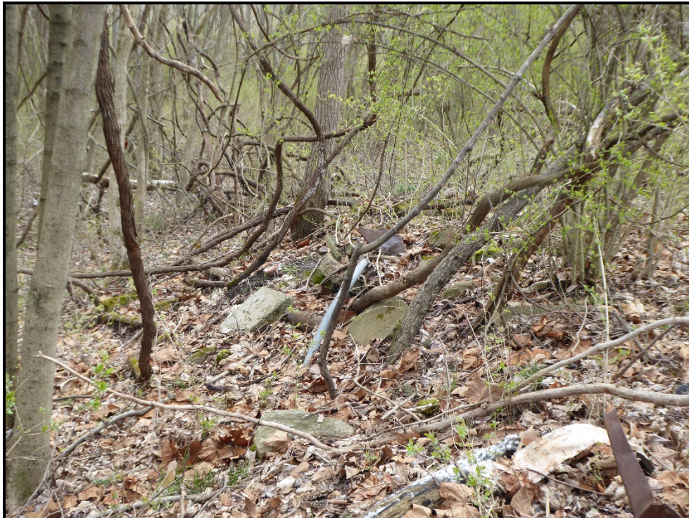
Figure 32: Rubble pile on slope northeast of foundation, facing east.
