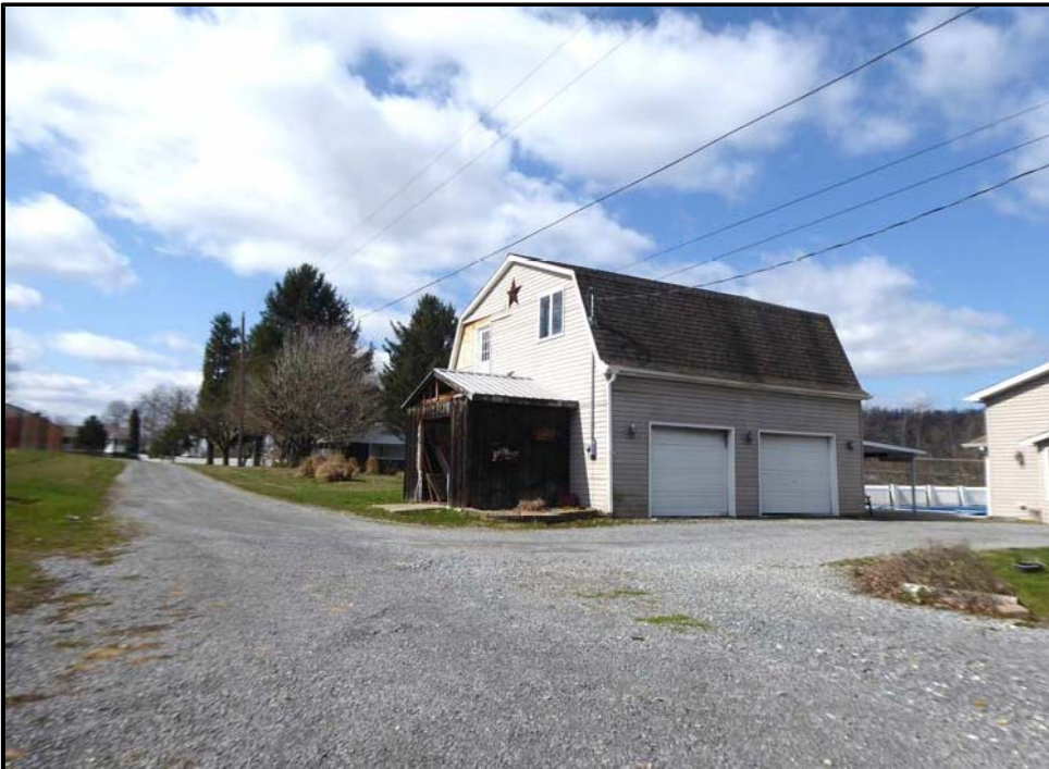
Photo 16: Garage at 3734 Collins Ferry Drive, southeast (side) and northeast (front) façades, facing southwest.
