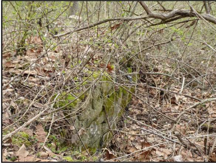
South foundation wall, facing southwest.
