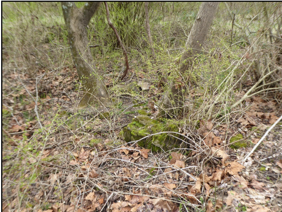
Figure 36: West foundation wall, facing south. Note interior portion of foundation in center of photograph.
