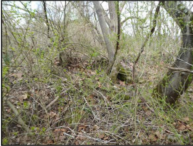
Foundation interior, facing west.
