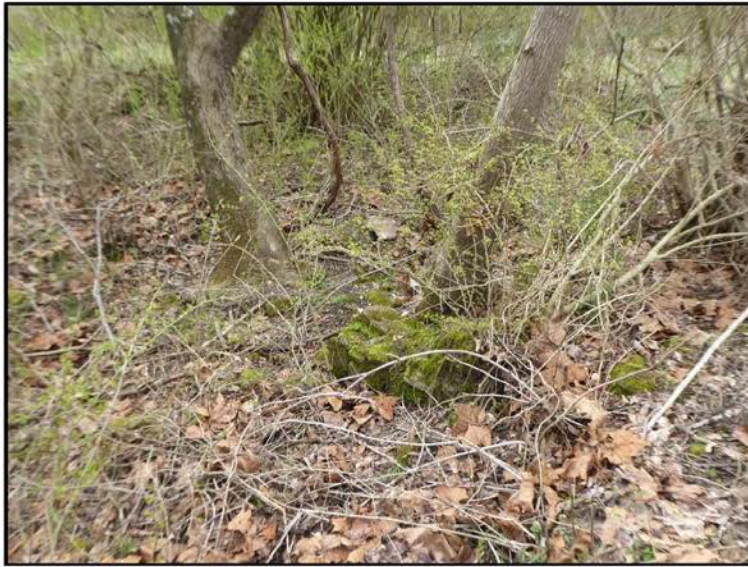
West foundation wall, facing south. Note interior portion of foundation in center of photograph.
