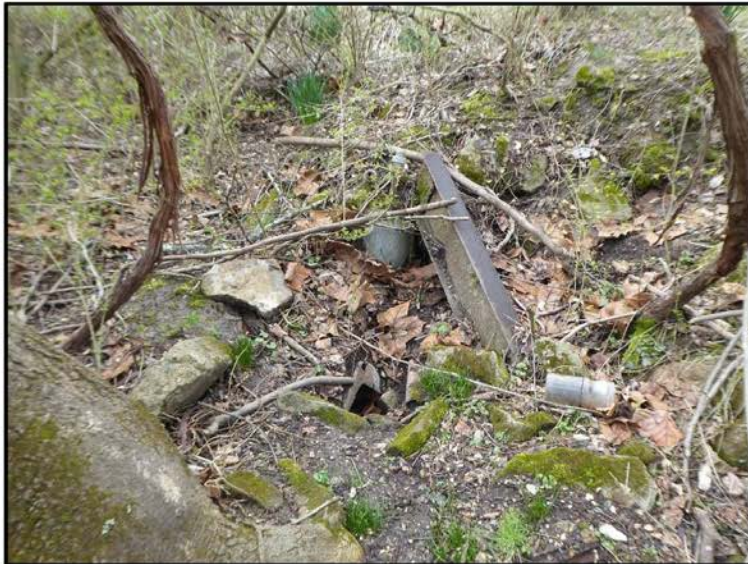
Rubble within the foundation.
