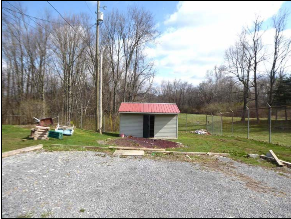
Photo 17: Outbuilding at 3734 Collins Ferry Drive, southwest (front) façade, facing northeast.
