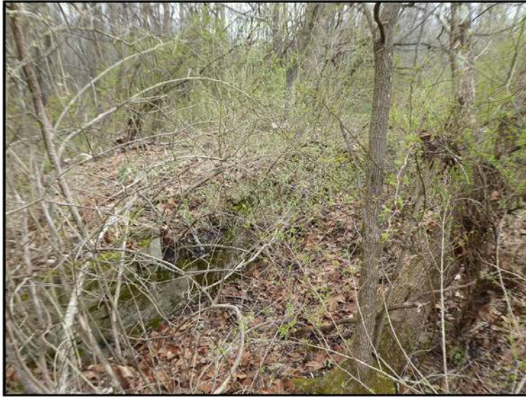
North foundation wall, facing northeast.
