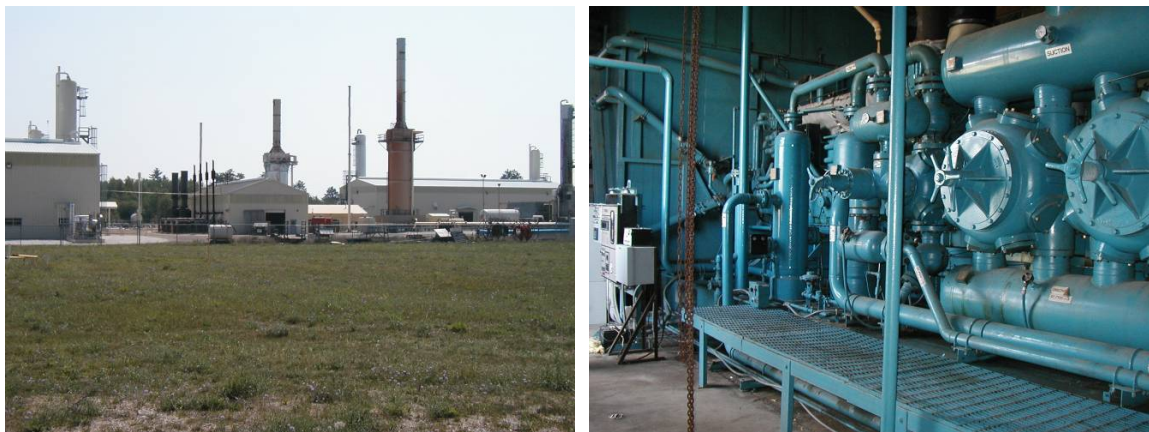
Figure 9.2. Gas compression and dehydration facilities at the northern Michigan candidate test site.
