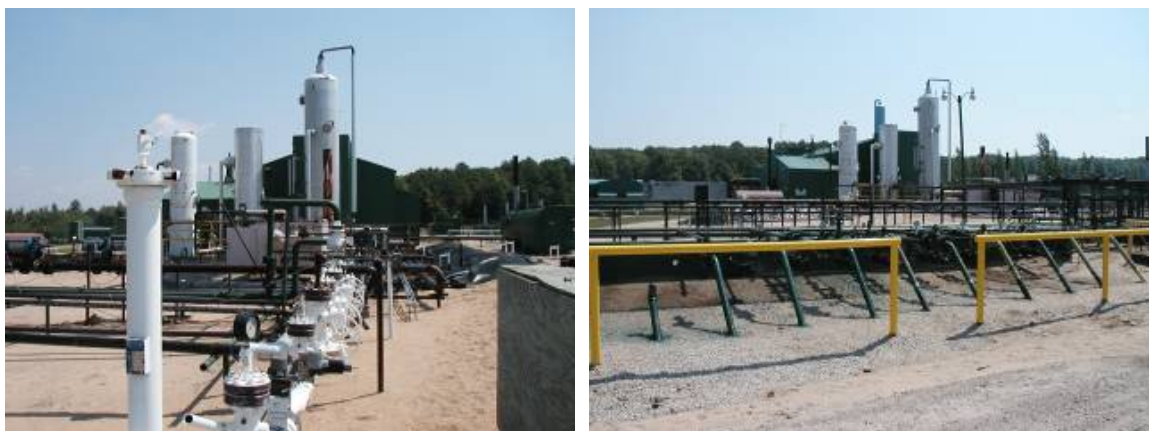
Figure 9.3. CO 2 pipeline feeding existing EOR wells at the northern Michigan candidate test site.
