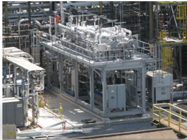
Existing MTR Membrane Module (20 TPD evaluated at NCCC)
