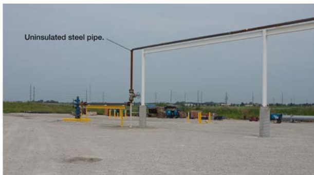
Configuration of pipeline near wellhead (no insulation)
