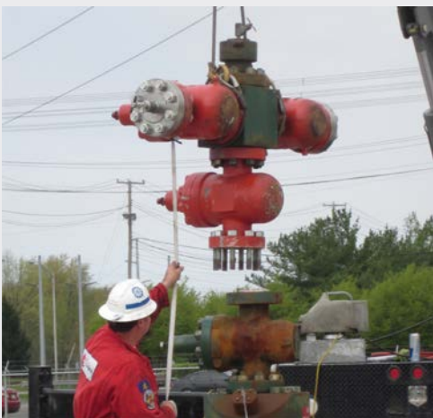
Replacement of the Wellhead Valve Assembly on One of the Injection Wells during the Post-Injection Monitoring and Maintenance Period
