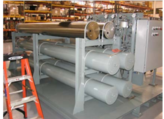
Assembly of skid-mounted pressurization system in progress (left and right sides)
