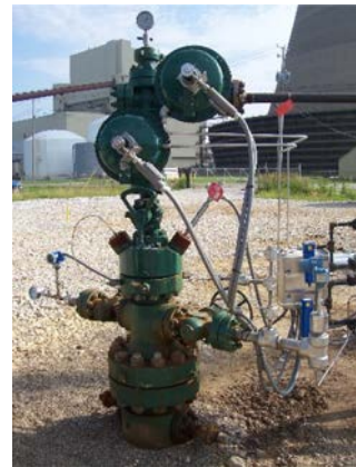
½-inch diameter stainless-steel line connecting well annulus to pressurization system
