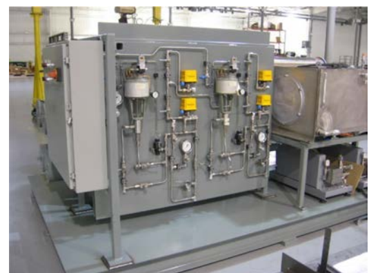
30-gal accumulator tanks for annular fluid (top right) and four 35-gal cylinders for nitrogen (middle bottom right)
