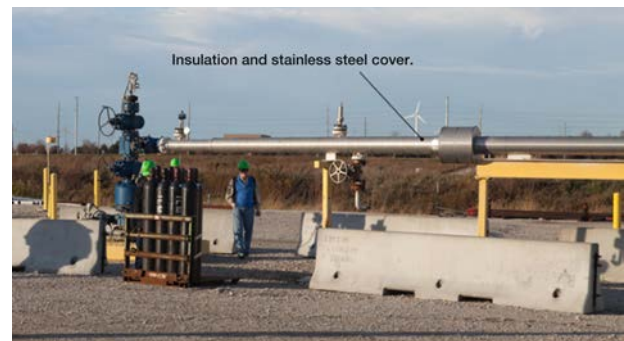
Insulated pipeline at wellhead
