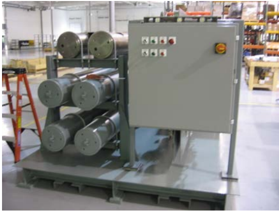
Fluid system valves mounted on skid (Nitrogen system valves are monitored on back side and not visible in this photo)
