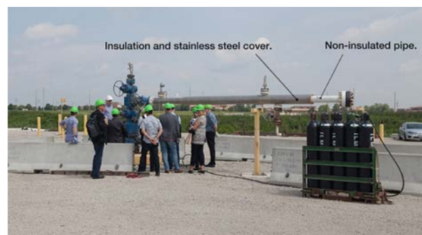
Partial insulation of pipeline during construction
