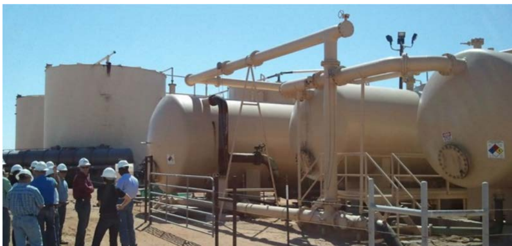
Figure E-2: Image of multiple production separators
