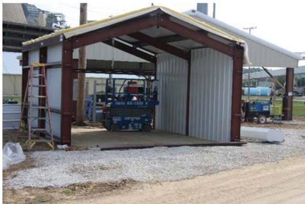
Building for housing annular pressurization system under construction
