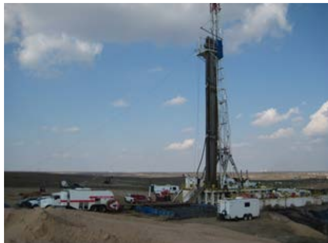
FIGURE 9. CHARACTERIZATION WELL BEING INSTALLED IN THE WELLINGTON FIELD IN SUMNER COUNTY, KANSAS.
