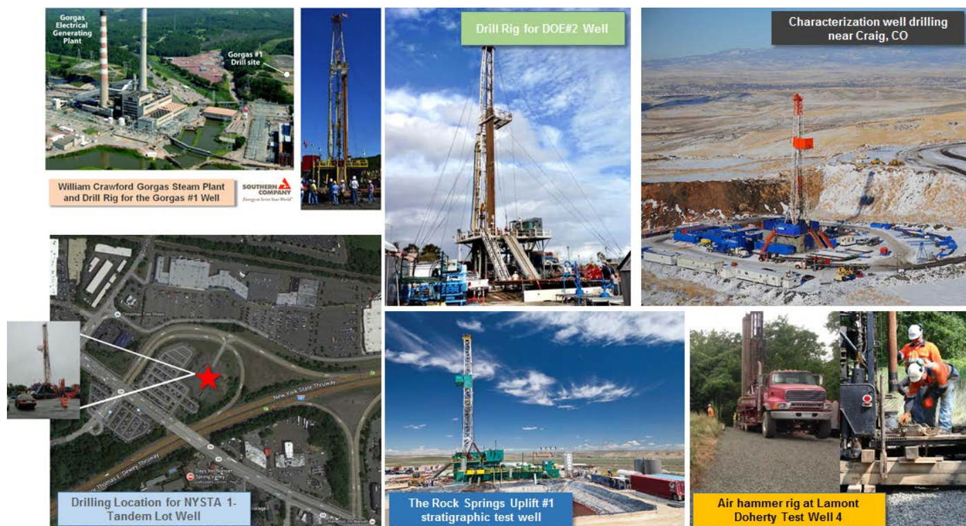
FIGURE 5. DRILLING OPERATIONS AT VARIOUS ARRA SITE CHARACTERIZATION PROJECT SITES. THE IMAGES CORRESPOND TO DIFFERENT PROJECT SITES DRILLING NEW WELLS. TOP LEFT (UNIVERSITY OF ALABAMA), BOTTOM LEFT (SANDIA TECHNOLOGIES), TOP MIDDLE (GEOMECHANICS TECHNOLOGIES), BOTTOM MIDDLE (UNIVERSITY OF WYOMING), TOP RIGHT (UNIVERSITY OF UTAH), AND BOTTOM RIGHT (SANDIA TECHNOLOGIES).
