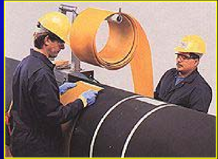
Clock Spring Installation
