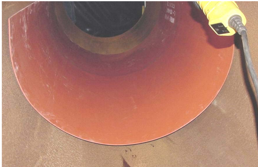
Figure 60 - Rubber Sheet Protecting Inflatable Bladder From Epoxy for Test 08
