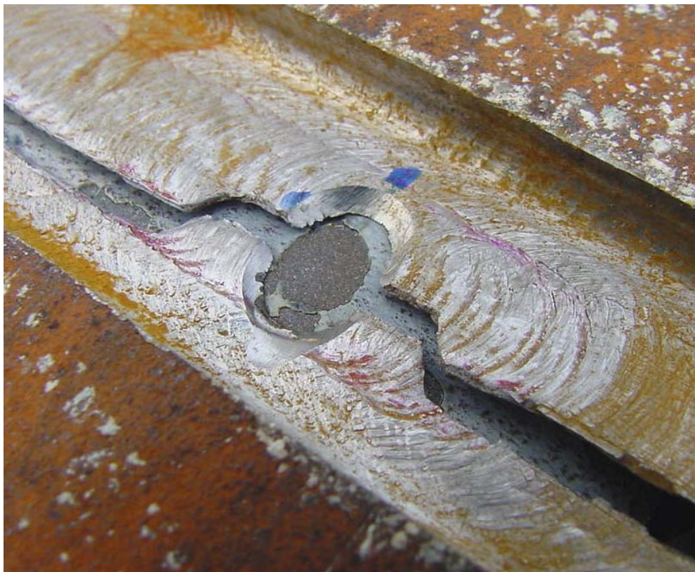
Figure 174 - Close Up of Test 13 Damage after Burst Test
