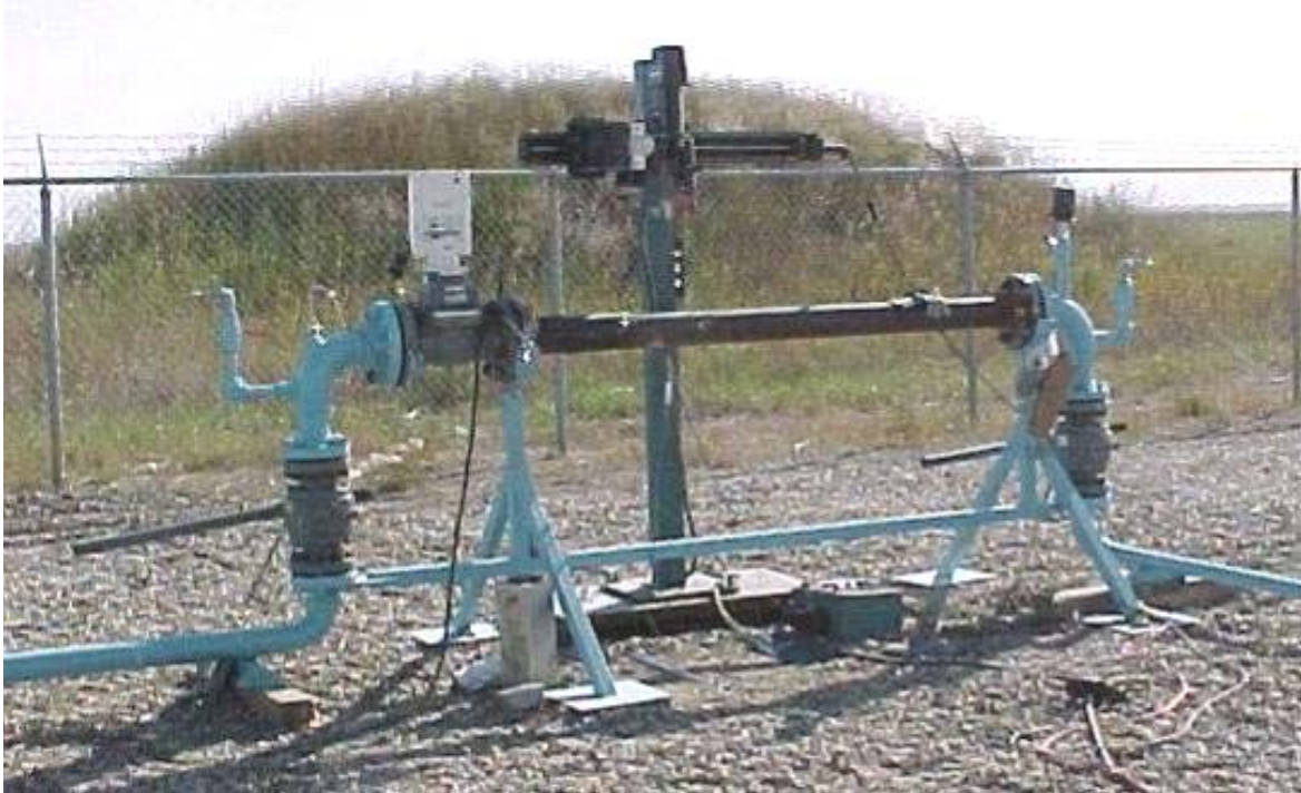
Figure 131 - Set-Up for Welding Thin Wall Pipe with Pressurized Methane Gas
