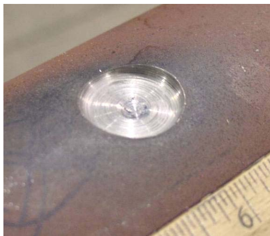
Figure 15 - Short/Deep Simulated Corrosion Damage for 114.3 mm (4.5 in.) Pipe
