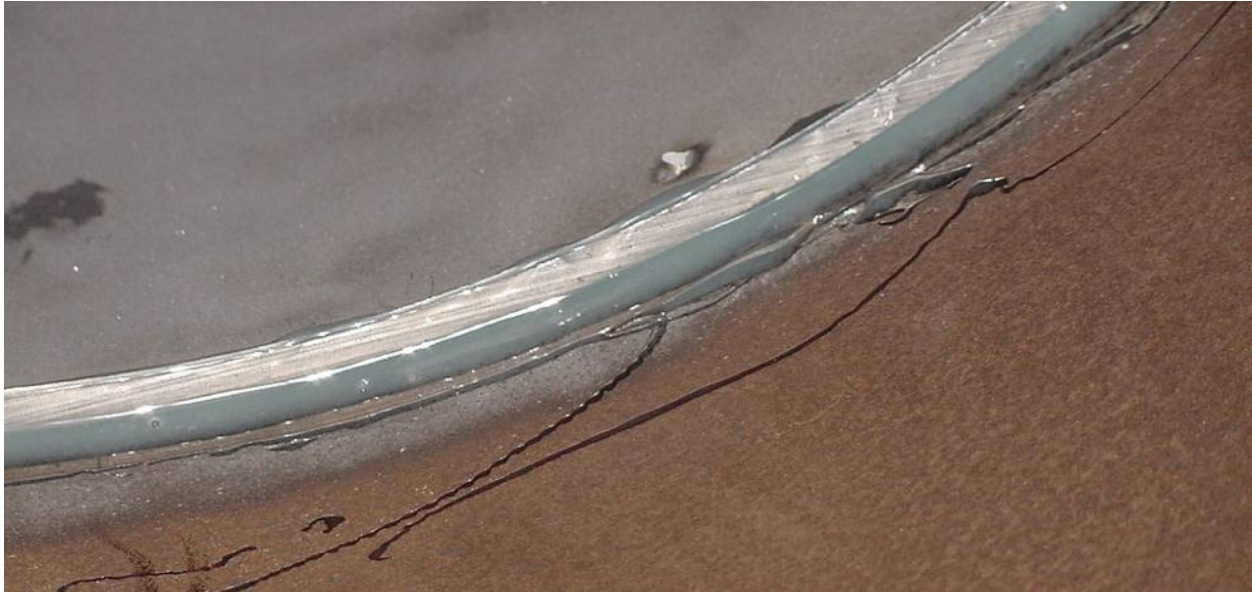
Figure 59 - Test 08 Steel Patch Prior to Epoxy Curing (Circumferential Fillet)
