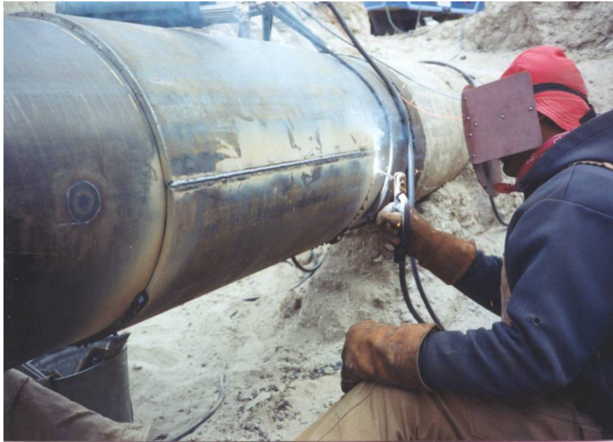
Figure 1 - Installation of a Full-Encirclement Repair Sleeve
