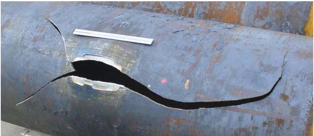
Figure 97 - 558.8 mm (22 in.) Pipe with Un-Repaired Damage After Burst Testing
