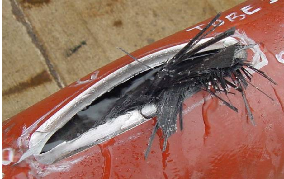
Figure 146 - Test 02 Pipe with GF Liner Repair of Long/Shallow Damage After Burst Test
