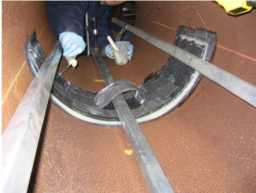
Figure 45 - Clamping Bars Used to Hold Test 04 CF Patch in Place
