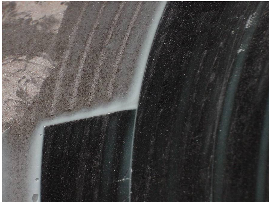
Figure 166 - Close Up of Completed Helically Wound Steel Strip Repair
