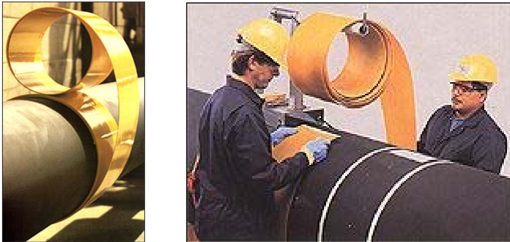
Figure 7 - Clock Spring® Fiber-Reinforced Composite Device for Pipeline Repair
