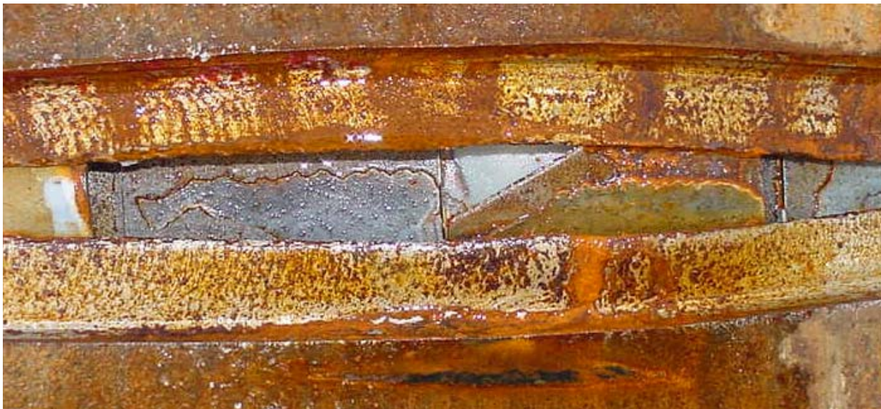
Figure 177 - Close Up of Test 14 Damage after Burst Test
