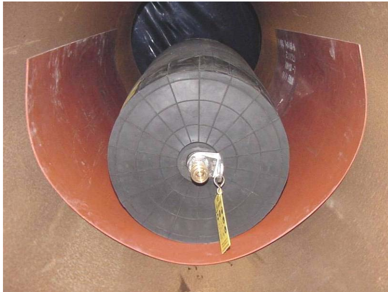
Figure 61 - Bladder Prior to Pressurization for Test 08
