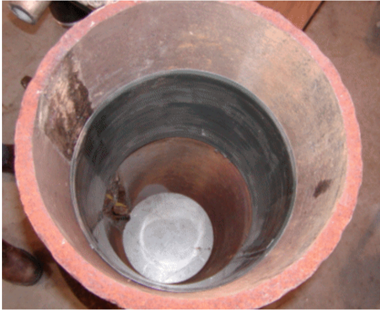
Figure 10. Successfully Installed Repair Sleeve
