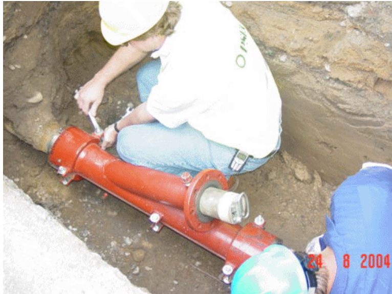
Figure 59. Attaching 4-in. Entry Fitting to Pipe Prior to Welding
