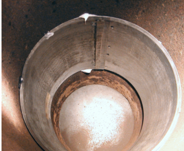
Figure 56. Successfully Patched Joint
