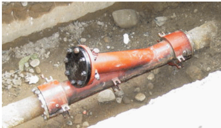
Figure 64. 4-in. Entry Fitting Ready for Burial
