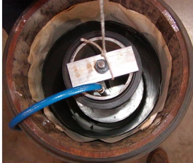
Figure 19. Bladder/Patch Assembly Hung in Joint
