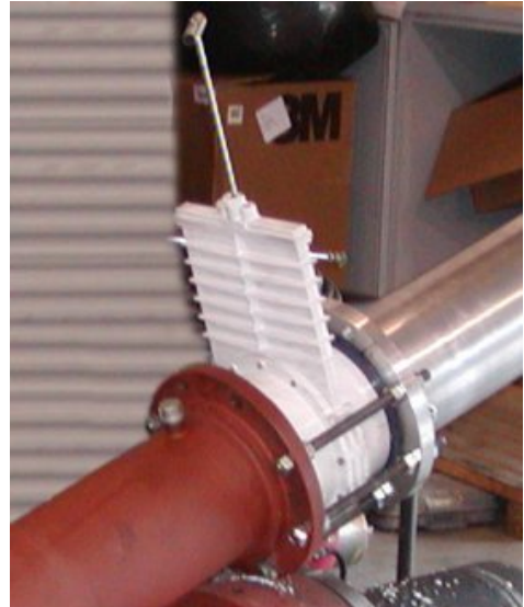
Figure 41. PVC Control Valve
