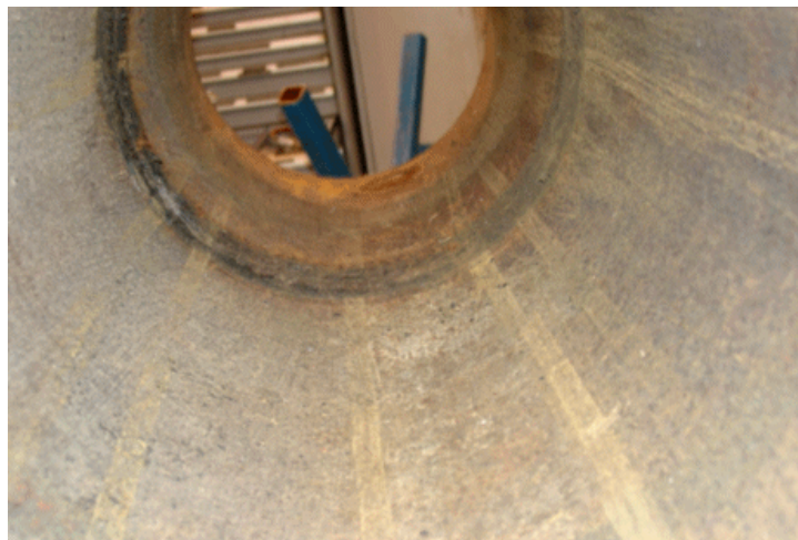
Figure 9. Cast-Iron Pipe ID after Cleaning
