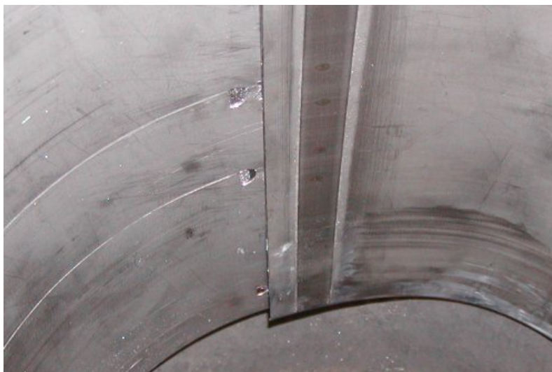
Figure 20. Partial Ratchet Engagement After Patch Setting
