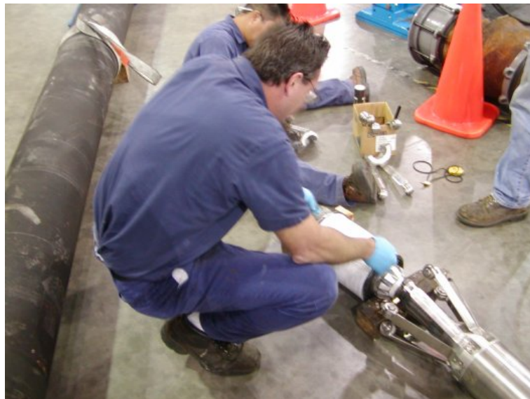
Figure 55. Installing Patch onto Inflation Bladder
