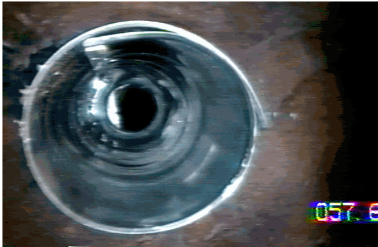
Figure 63. Partially Engaged Patch at 57.6 ft
