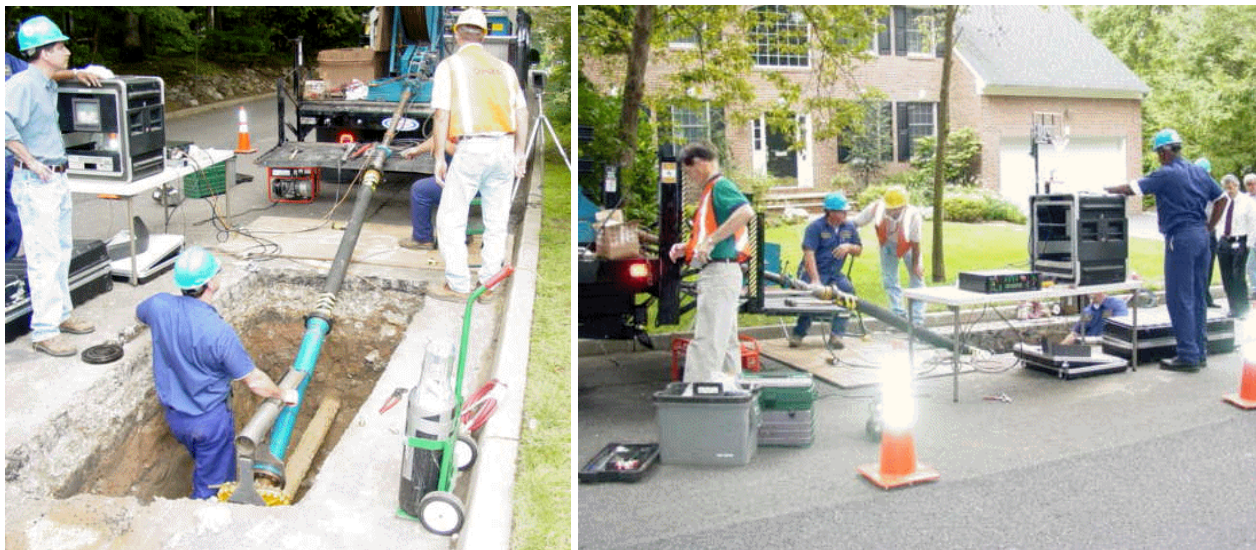
Figure 58. Field Test Site for Small-Diameter System
