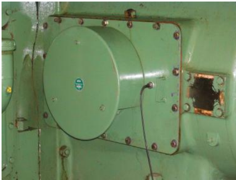
Figure 3-15. Cable from RLM Antenna (GMW10; Williams Sour Lake Station; August 2003)
