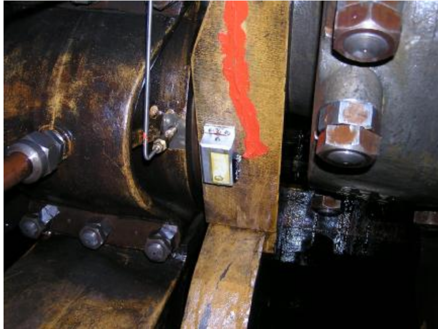
Figure 6-3. Strain Data Capture Module and Combined Power and Compressor Throw (Williams Station 60; February 2004)
