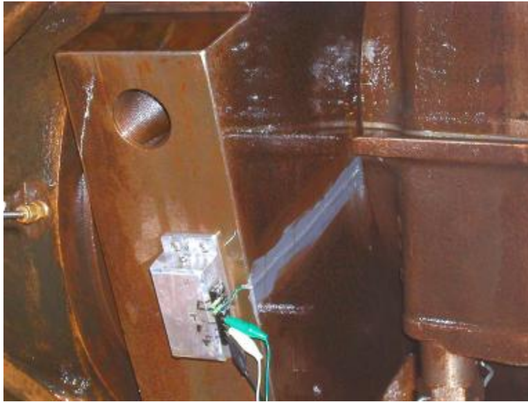
Figure 3-11. Strain Data Capture Module Installed (GMW10; Williams' Station 40 (Sour Lake); August 2003)
