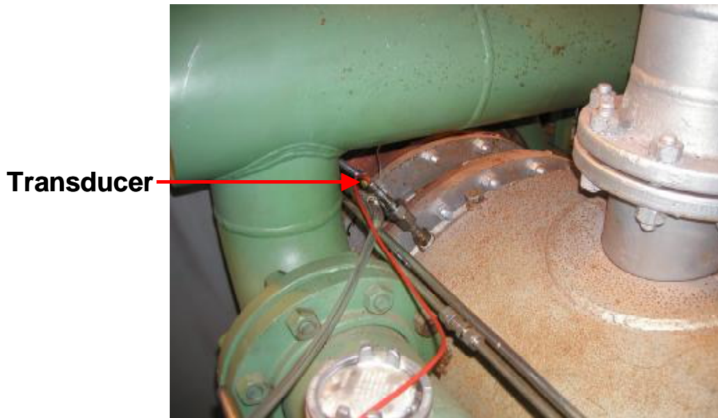
Figure 3-7. Pressure Transducer in Exhaust Manifold (GMW10; Williams Sour Lake Station; August 2003)
