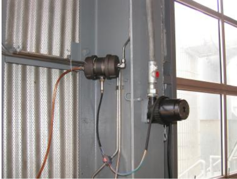
Figure 3-13. O 2 /NO x Sensor and Connection to Line from Stack (GMW10; Williams Sour Lake Station; August 2003)
