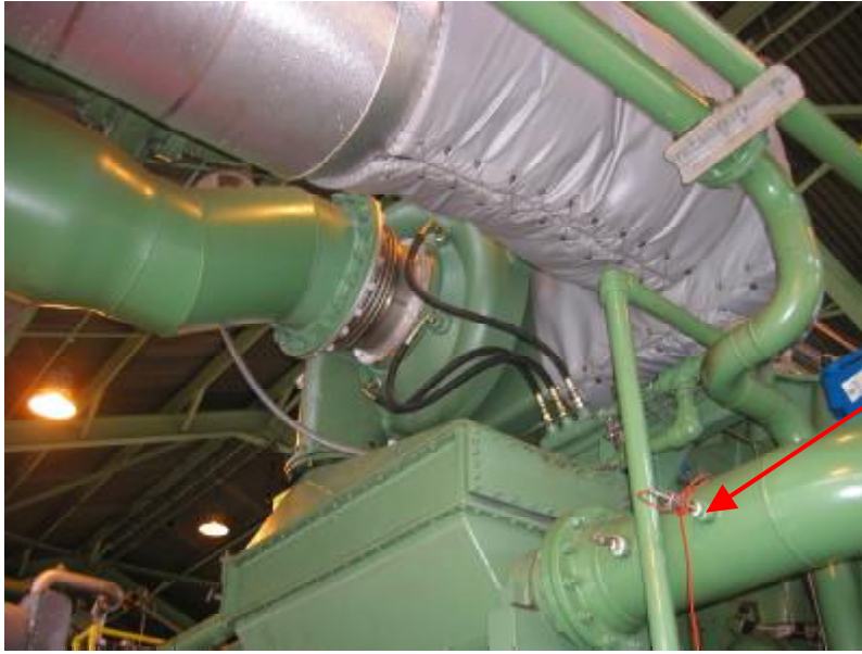
Figure 3-6. Pressure Transducer in Air Intake Manifold (GMW10; Williams Sour Lake Station; August 2003)
