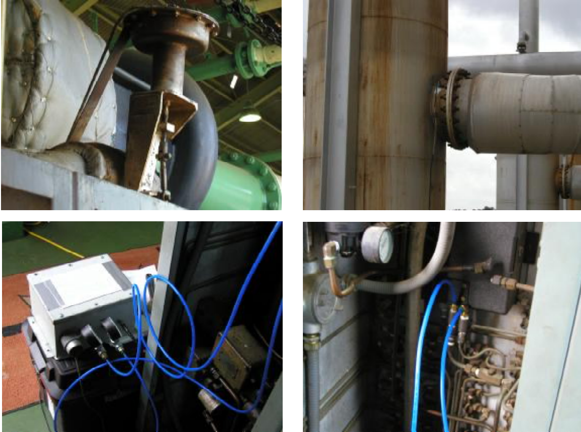
Figure 19. Elements of Wastegate Control for Equivalence Ratio
