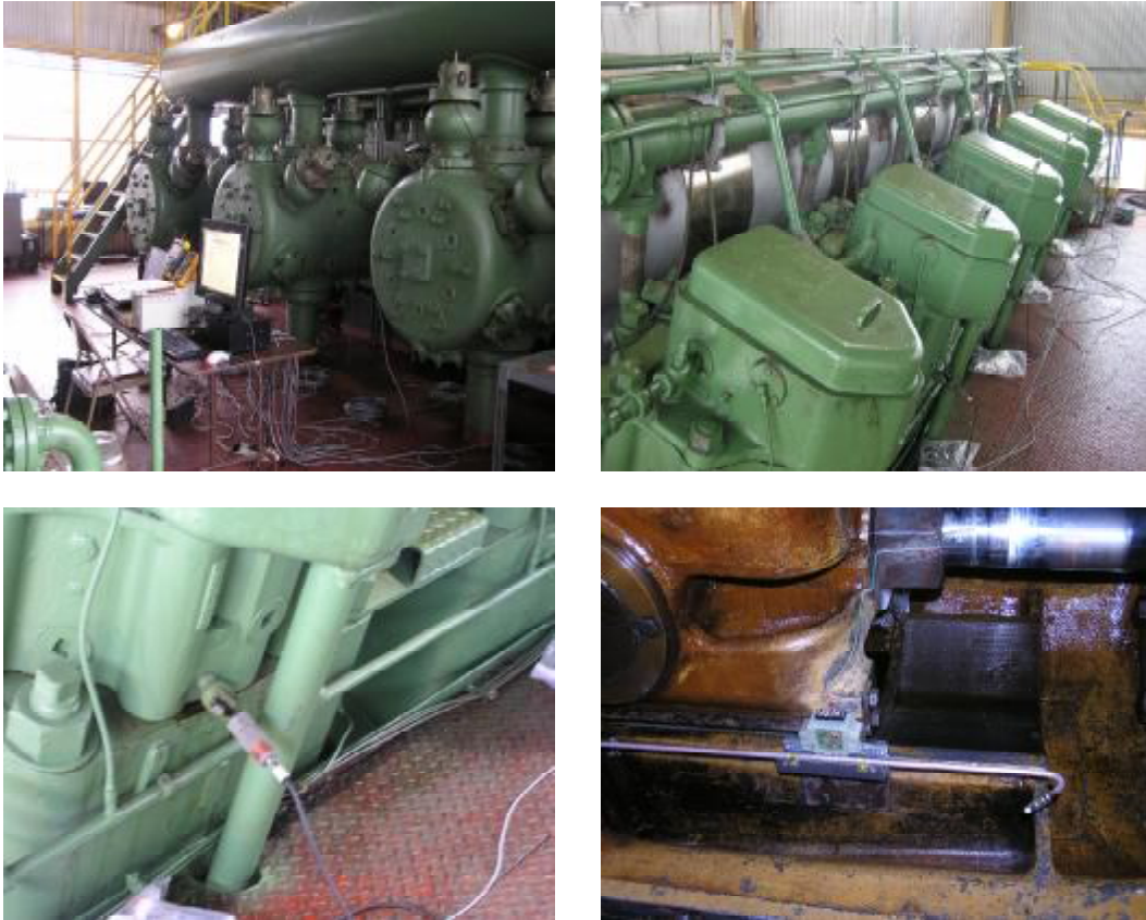
Figure 4. Williams Station 60; GMW10 - Unmodified
