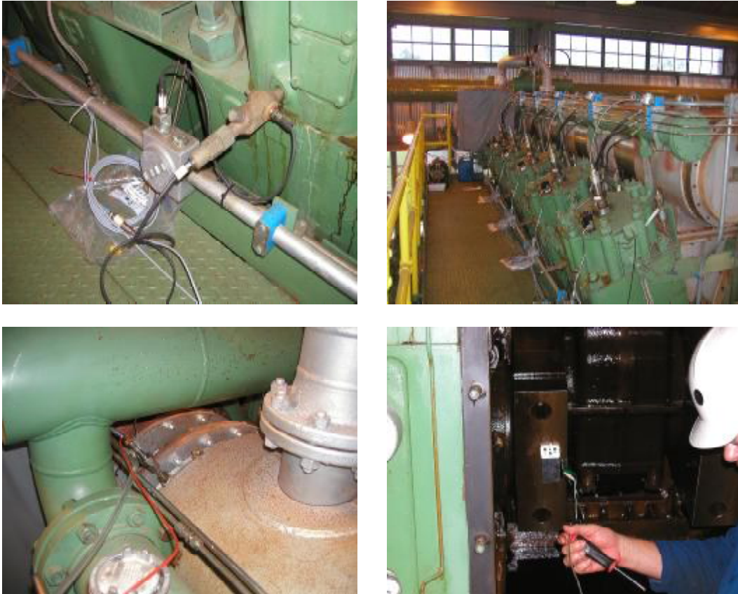
Figure 2. Williams Station 40; GMW10 with High-Pressure Fuel
