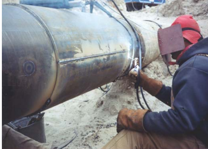
Figure 1 - Installation of a Welded Full-Encirclement Steel Repair Sleeve
