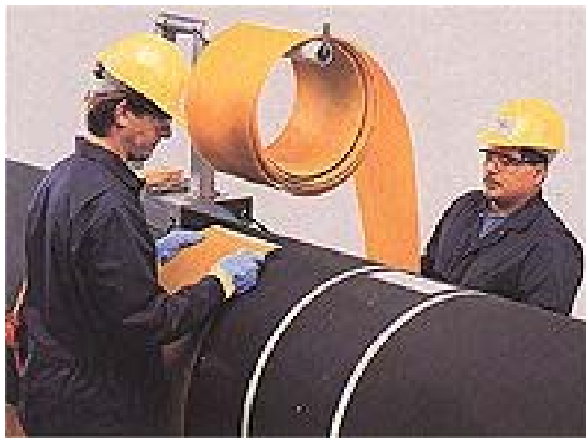
Figure 3 - Installation of a Fiber-Reinforced Composite Repair Device
