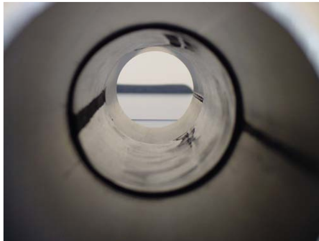
Figure 6 - Liner Inserted into Center of 4.5-in.-Diameter Pipe
