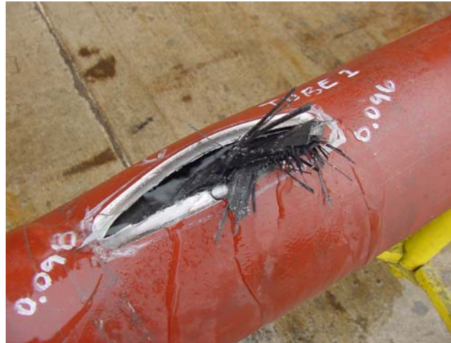
Figure 7 - Pipe Section with Liner Following Hydrostatic Pressure Test
