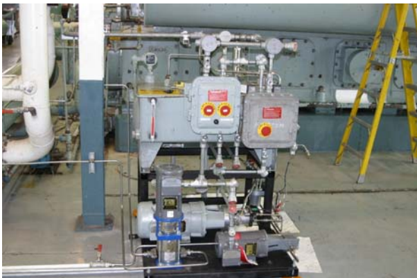
Figure 36 - Pump Cart & Diesel Tank
