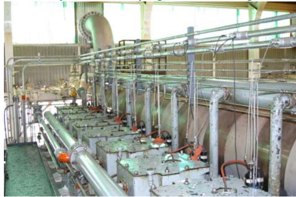
Figure 35 - SUTC power Cylinders after RMI
