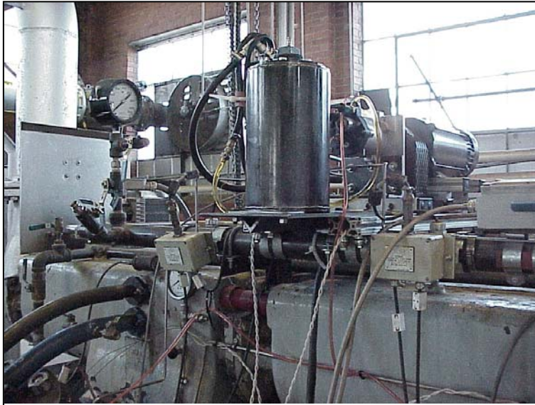
Figure 10 - Pilot fuel pump, storage, filter
