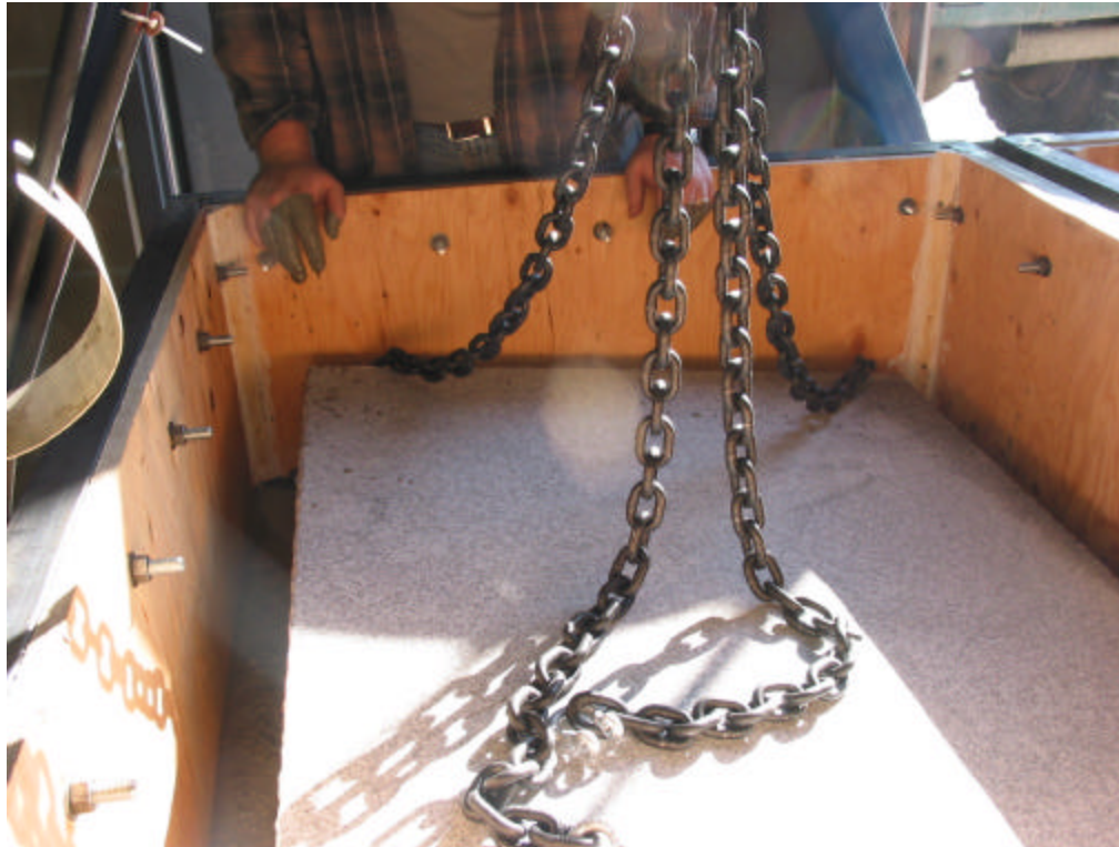
Figure 6: Positioning granite block at 10° angle before concrete pour
