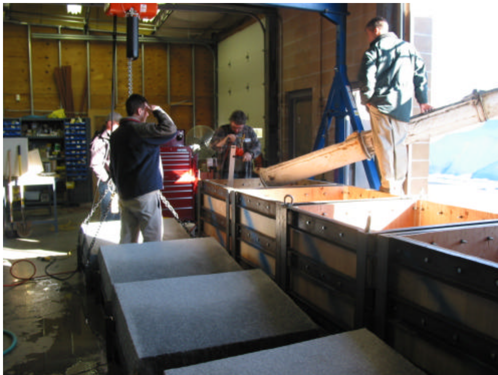
Figure 7: Pouring concrete for first block
