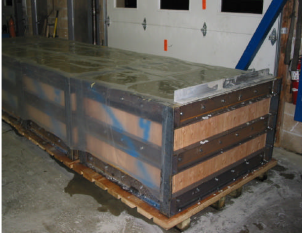
Figure 8: Finished blocks begin setting process
