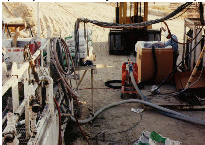
Figure 12. LWSA Field Test Mixing System
