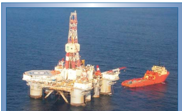
Figure 2. An offshore platform in the Gulf of Mexico. (Photo by J. Veil, Argonne National Laboratory)
