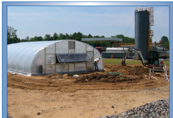
Figure 4. Construction of the demonstration-scale wetland system built to evaluate onsite performance for treatment of actual gas storage-produced waters. The wetland is enclosed in a greenhouse.
