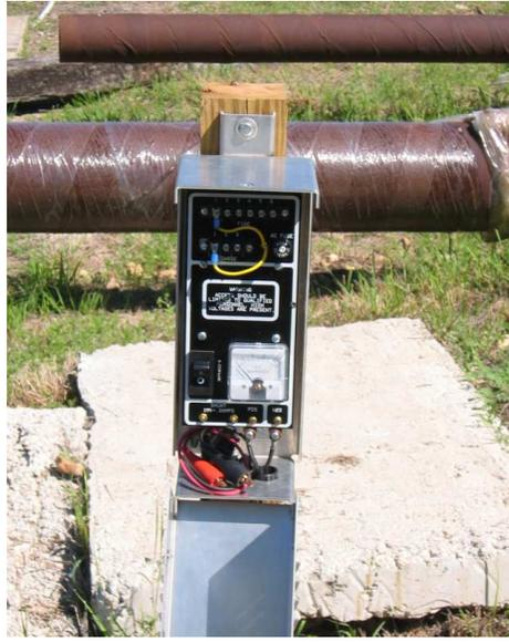
**Figure 18. Details of CP rectifier installation**
