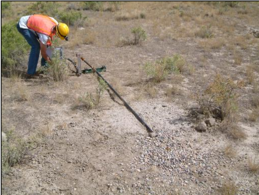
Site 4 – Underground leak emitting through gravel.
