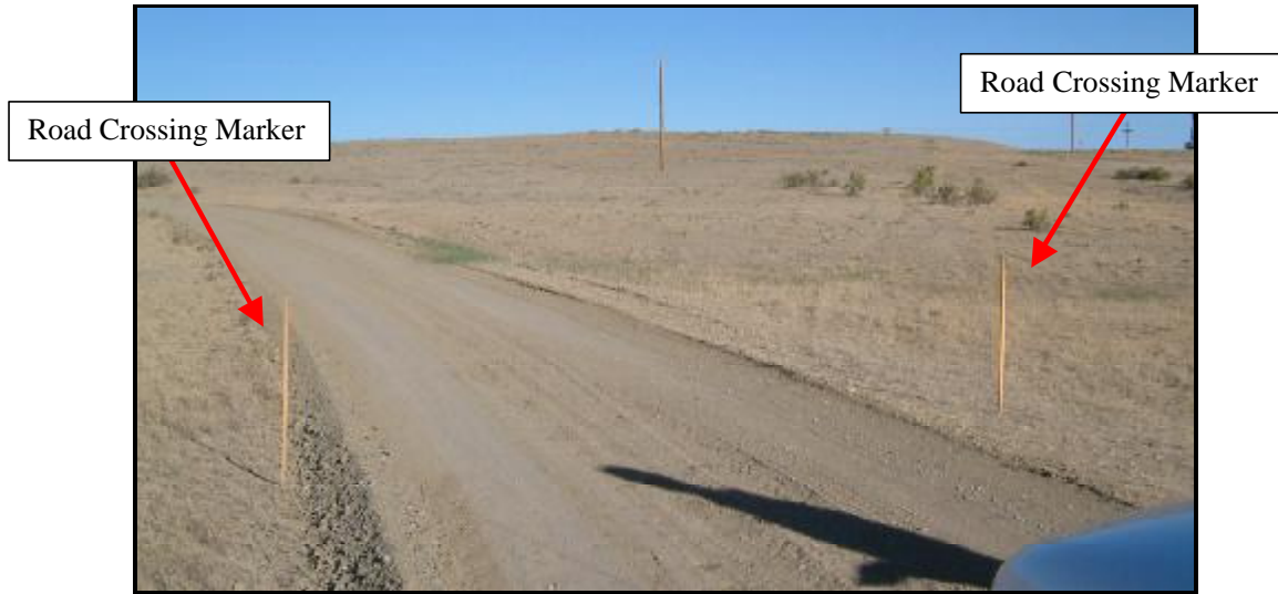
Figure 3.2 Road Crossing Marker
