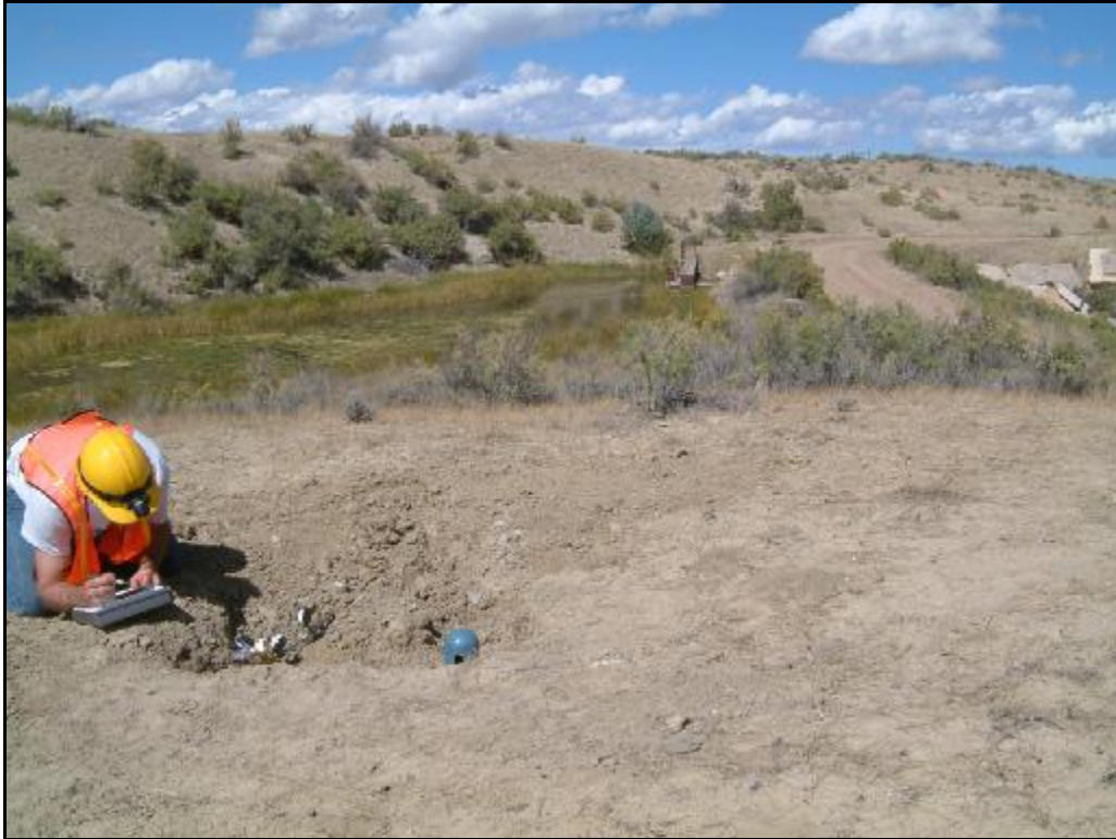
Site P5 – View of site and vegetation. The leak emits beneath the greasewood bushes in the middle of the picture.
