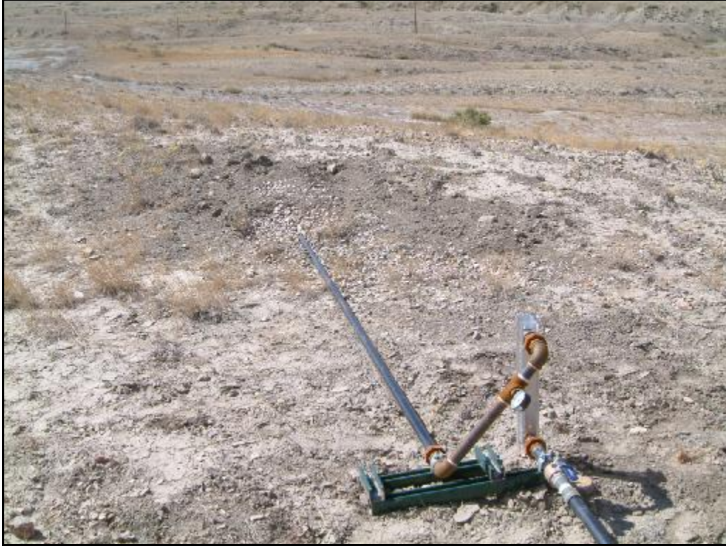
Site 6 – View at the top of the hill. Underground leak at gravel located approximately 10 feet from the rotometer.
