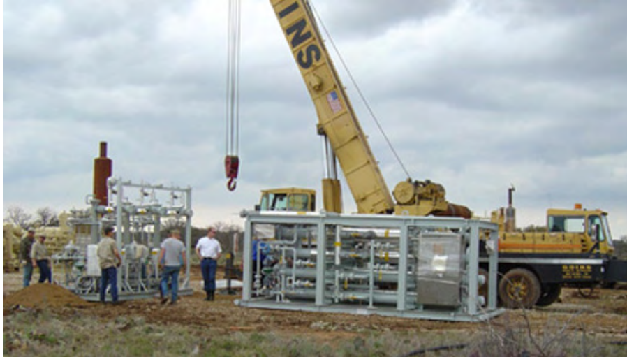
Figure 13. Membrane system being installed for NTE at Green Ranch, Texas.
