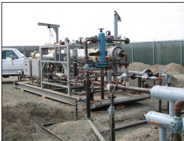
Figure 1. Skid-mounted nitrogen-separation membrane unit currently operating at a gas field demonstration site in Rio Vista, California.
