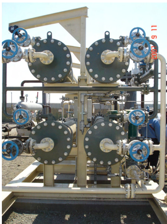
Figure 28. End view of commercial membrane system installed at Towne Exploration site in Rio Vista, California.
