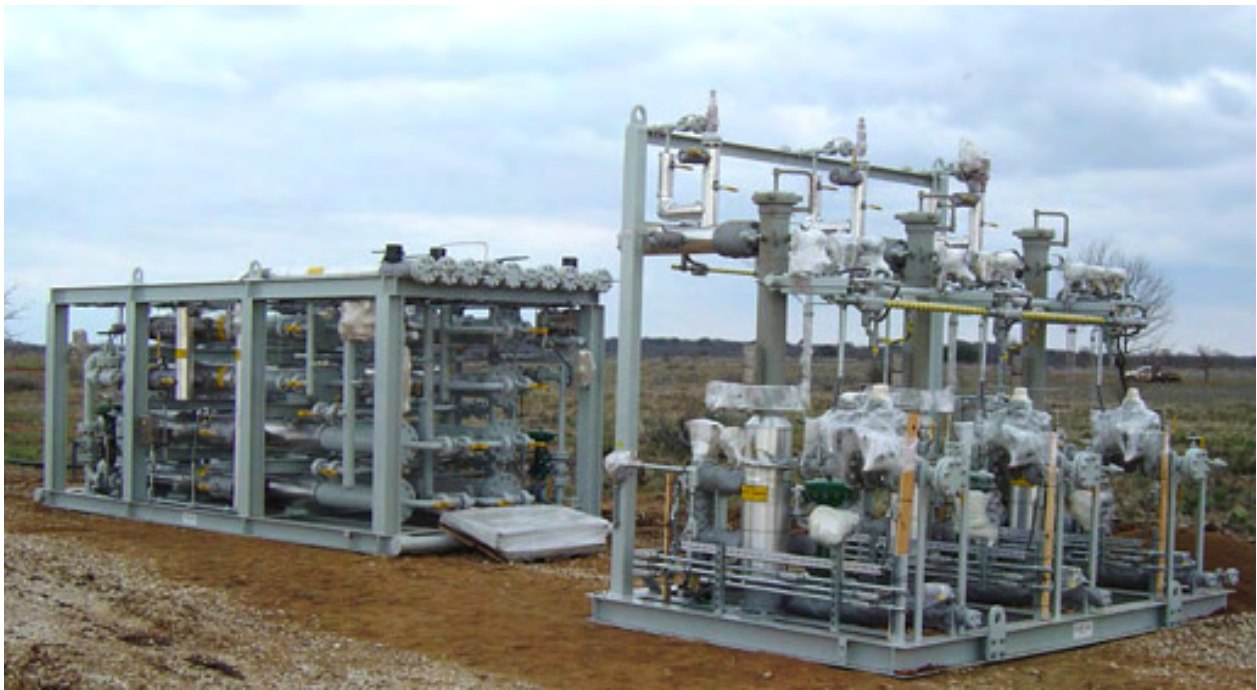
Figure 14. Membrane system being installed for NTE at Green Ranch, Texas.
