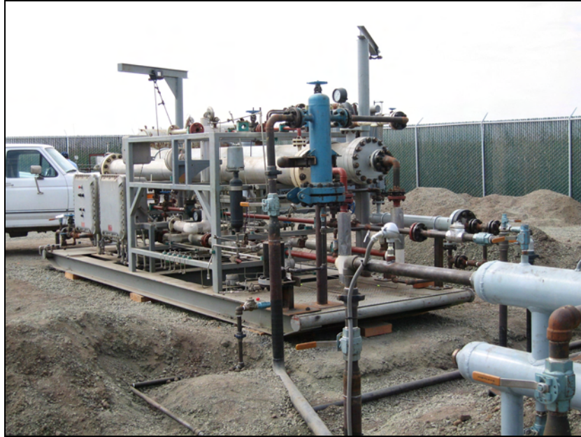
Figure 23. Skid-mounted nitrogen-separation membrane unit operated at a gas field demonstration site in Rio Vista, California. This was the most successful of the demonstration units for this project.
