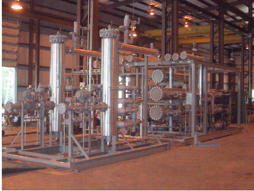
Figure 19. Syntroleum system ready for installation.
