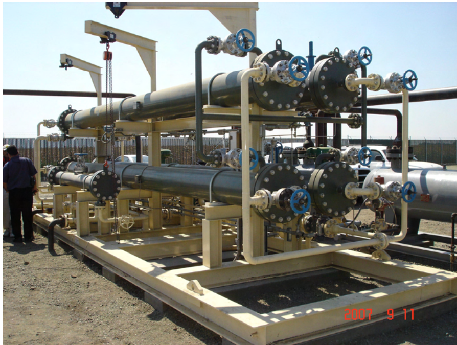
Figure 27. Commercial membrane system being installed at Towne Exploration site in Rio Vista, California.
