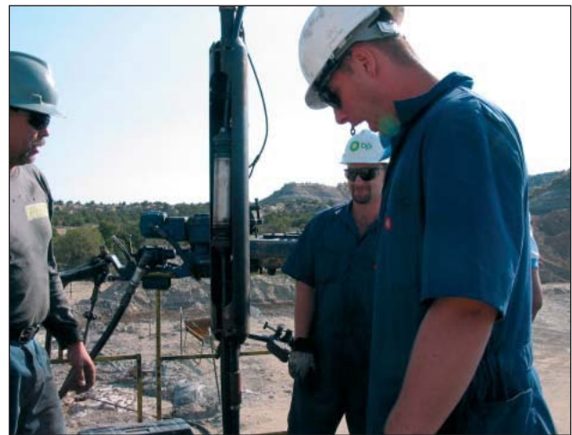
Figure 4 A geophone pod inside the geophone pod housing. The geophone pod housings are spaced 50 ft, and connected by two tubing joints.
