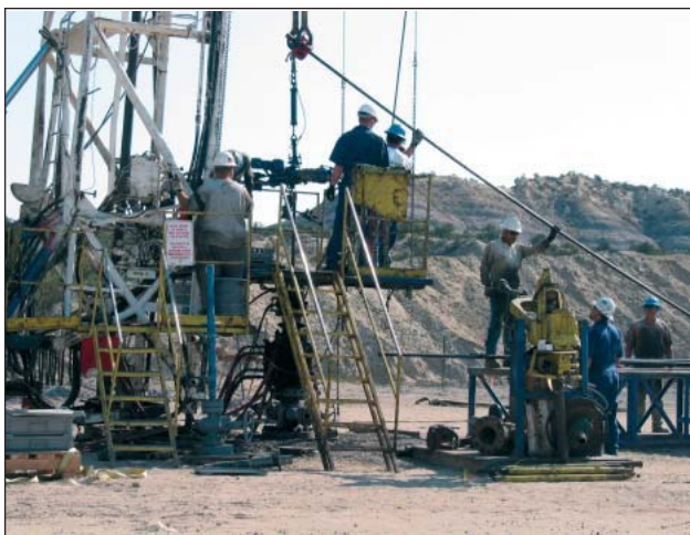
Figure 3 A work-over rig deploying the production tubing to which the downhole receiver array is attached.
